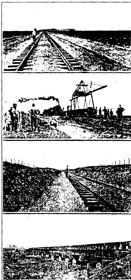
1—A long tangent in the flat country between Crane and Burns with eighty-foot fenced right of way. 2—Clyde tracklayer at work. 3—General Manager James W. Girard standing in the deepest cut on the line between Crane and Burns. 4—Trestle work was also light on this road.
