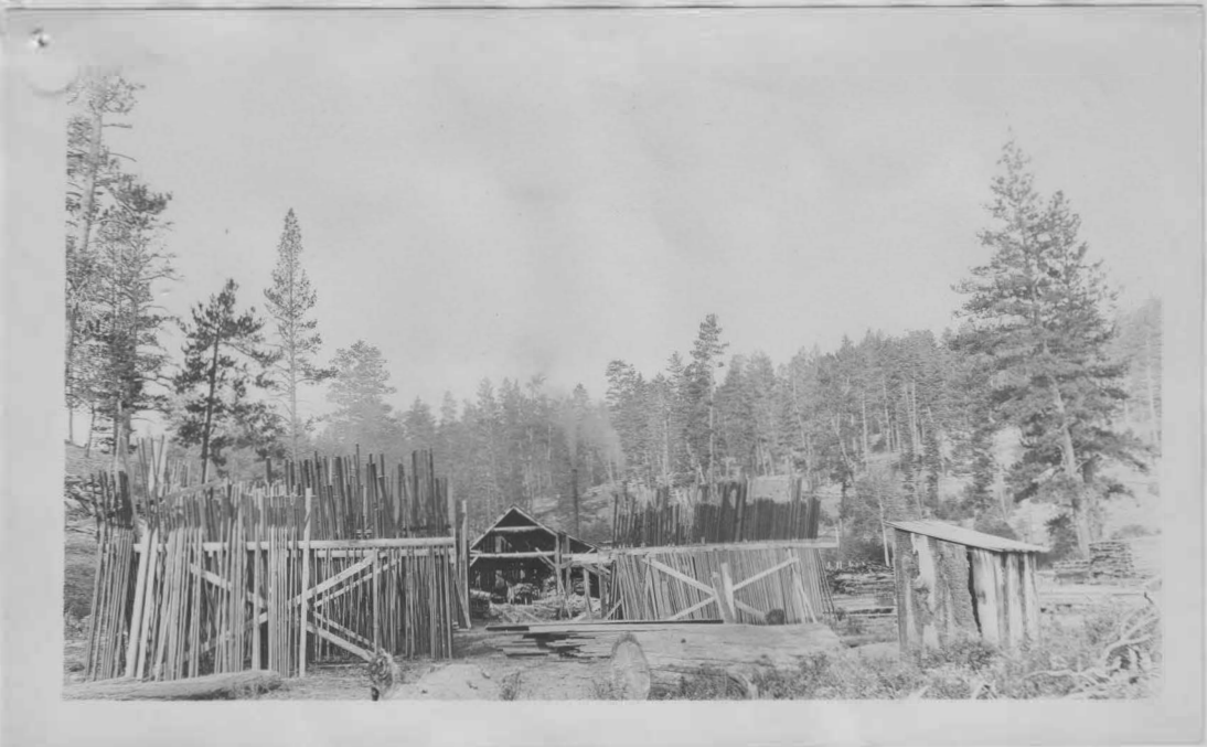
No. 16. Sawmill Plant showing mill, tramway, yard, and lumber racked for drying.
