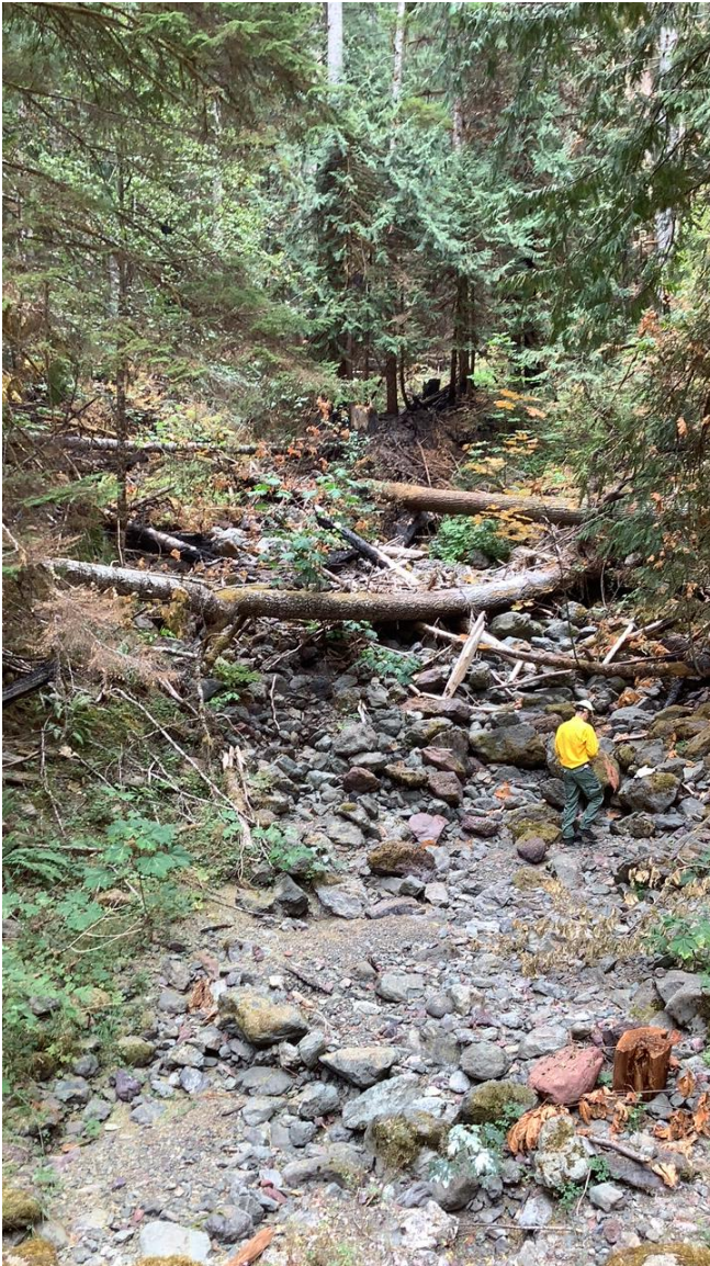
Photo 2 - Photo of the upstream channel where FSR 2451 crosses Copper Creek showing the range of clasts including large boulders and logs that can impact the functionality of the road-stream crossing infrastructure or be entrained in a debris flow and deposited downstream.
