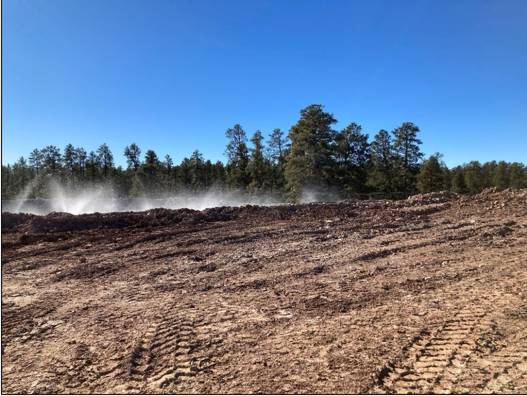
Photo 19 – Upper surface of development rock stockpile, facing SW. Hoses were online for dust abatement during site visit (Dec. 17)
