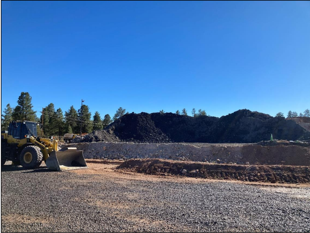
Photo 21 – Overlooking ore stockpile and loading ramp. (Oct. 28)
