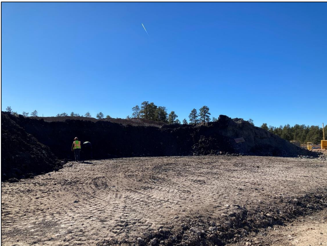
Photo 24 – Closer look at ore stockpile. (Dec. 17)
