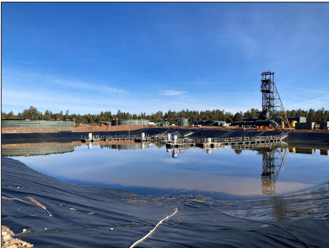
Photo 12 – Overlooking non-stormwater impoundment, facing NE. All evaporators were offline. (Nov. 25)
