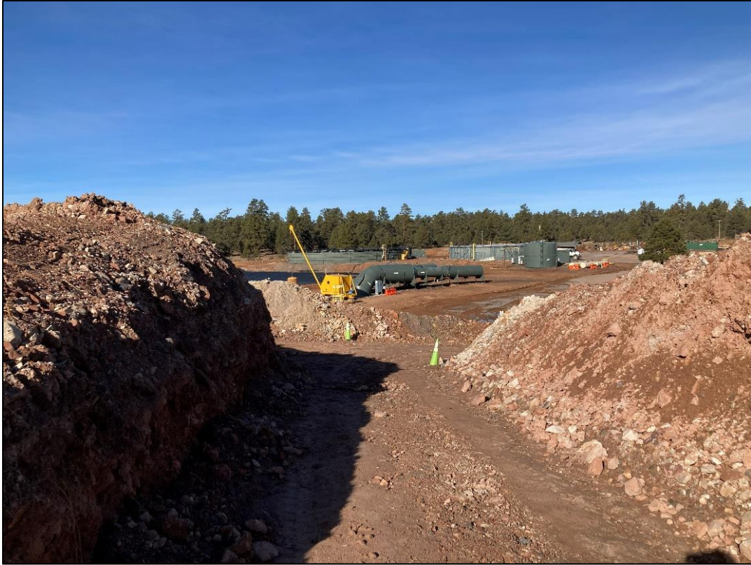
Photo 15 – Looking back at entrance of development rock stockpile. (Nov. 25)
