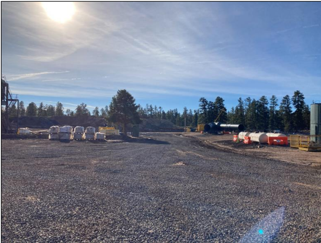
Photo 4 – Overlooking central mine area. Propane tanks and ventilation system on righthand side. (Nov. 25)
