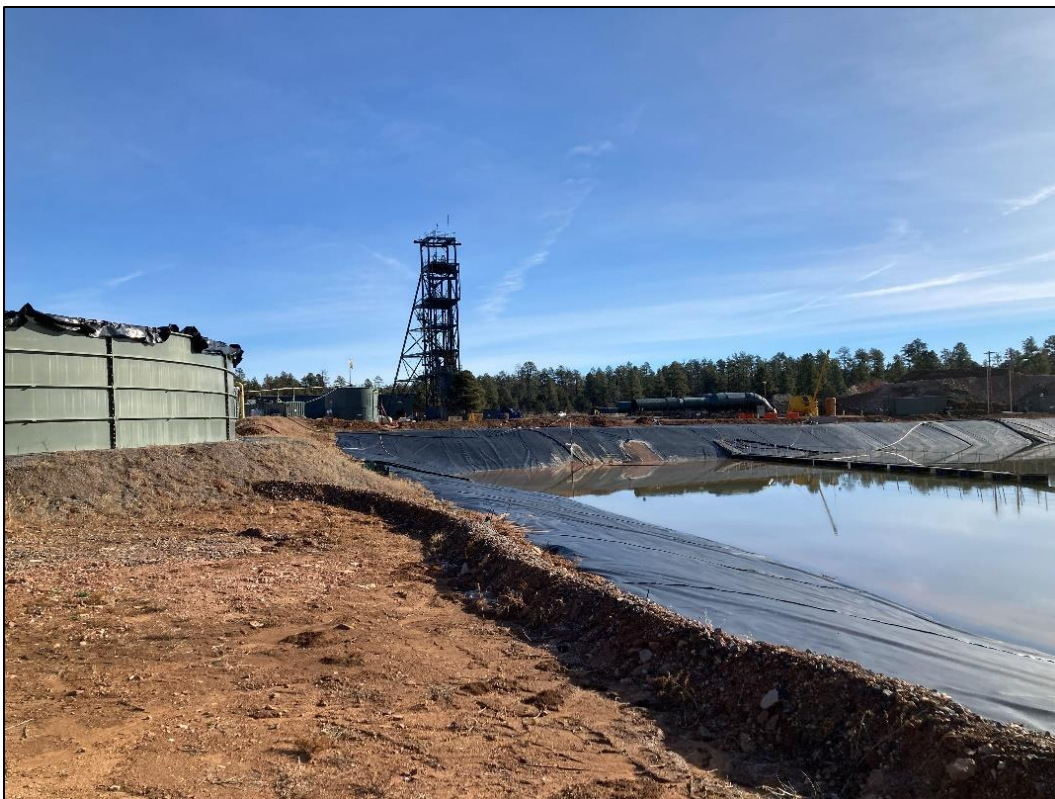
Photo 10 – Overlooking the safety berm adjacent to non-stormwater impoundment. (Nov. 25)
