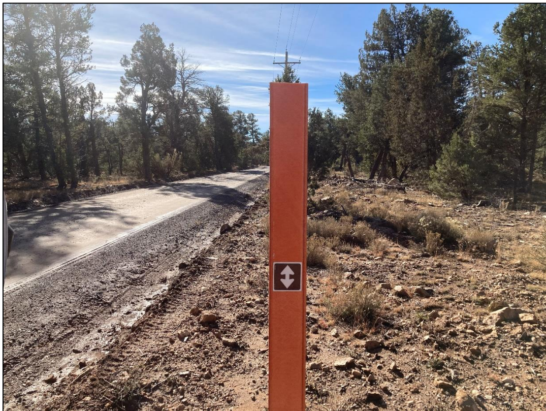
Photo 30 – Carsonite near the access route missing a sticker. (Nov. 25)
