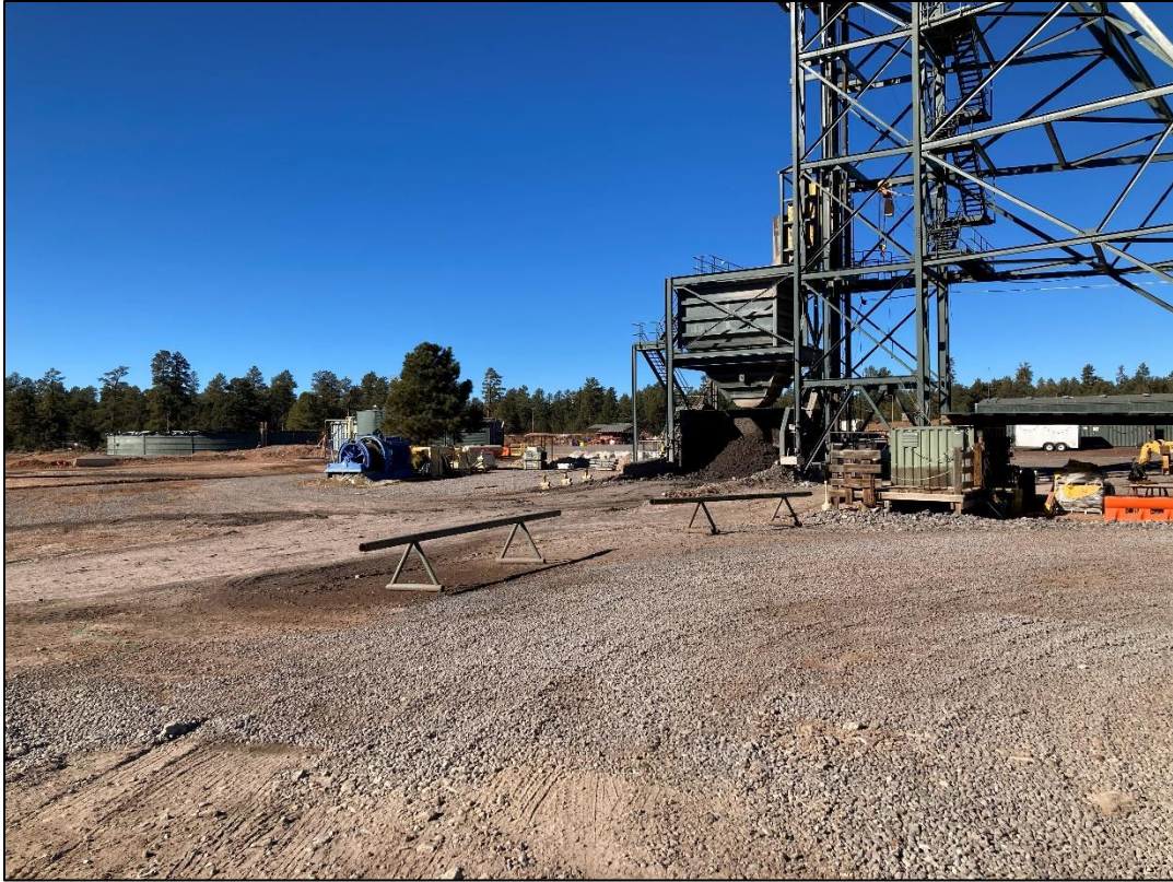
Photo 27 – Safety barriers near the ore hopper. (Dec. 17)
