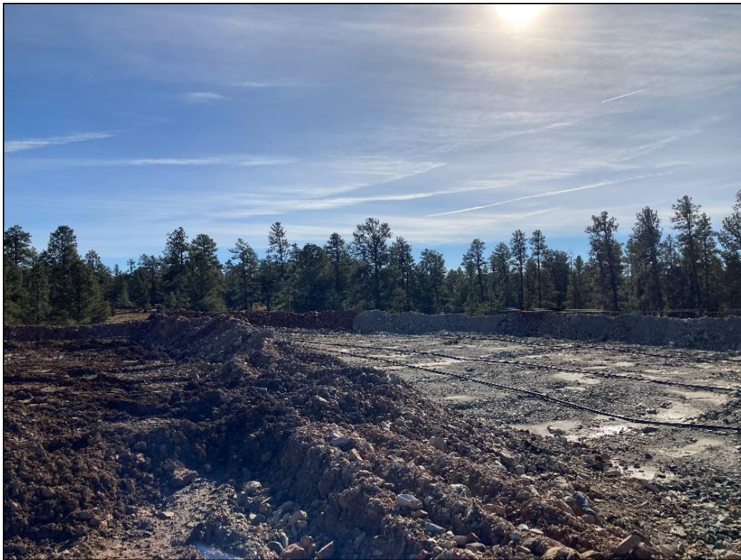
Photo 18 – Hoses used for dust abatement. (Nov. 25)
