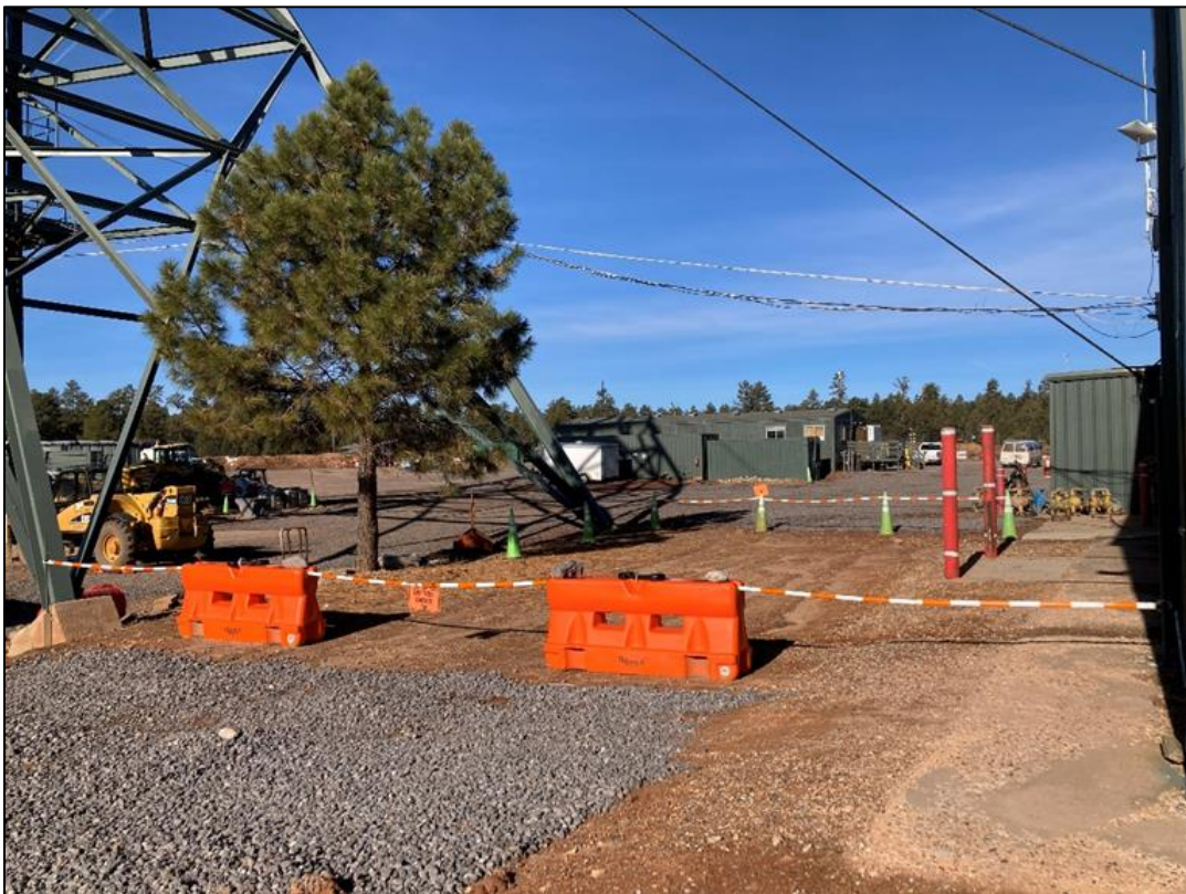
Photo 28 – Safety area between headframe and hoist room. (Nov. 25)
