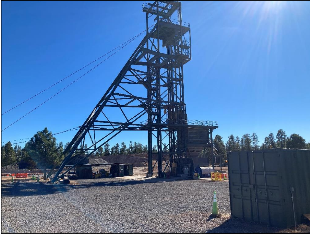
Photo 1 – View of the headframe from office trailer, facing south. (Oct. 28)
