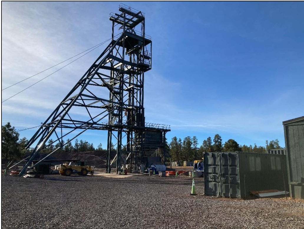
Photo 2 – Overlooking headframe, facing south. (Nov. 25)
