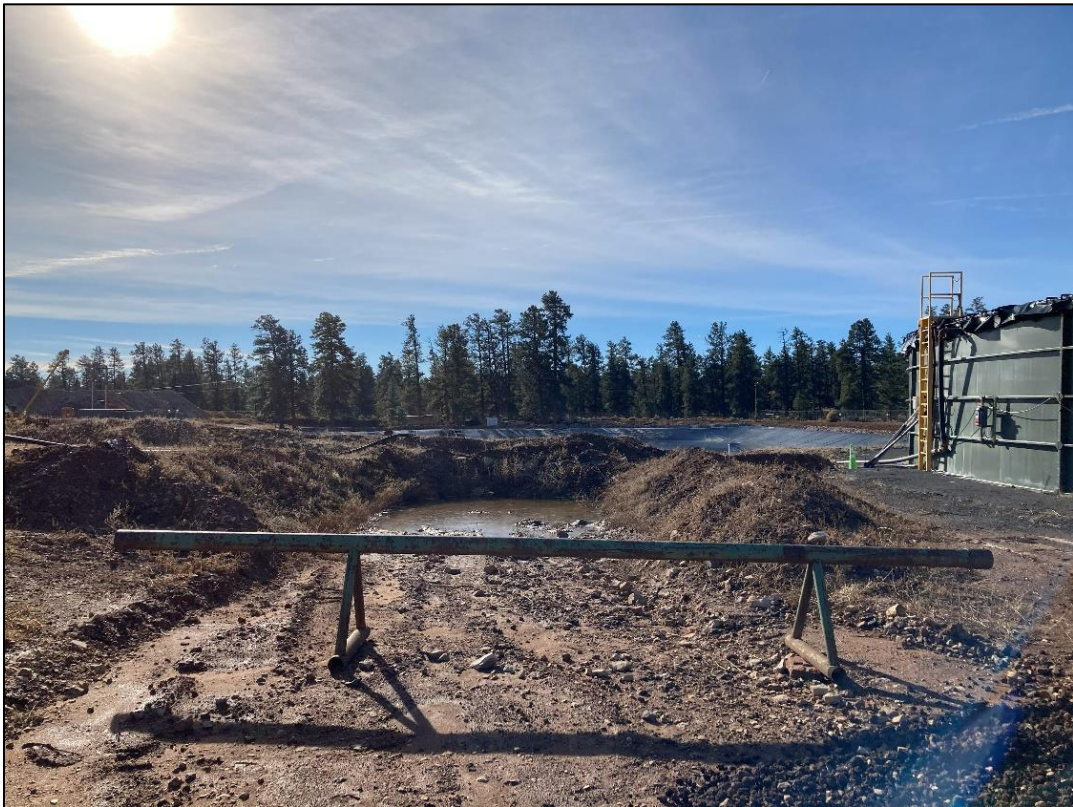
Photo 8 – Rainwater catchment from previous photo containing water. (Nov. 25)
