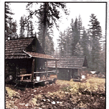
Figure 4: Shearer Guard Station.
