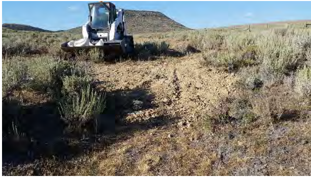
Figure 23. Back-filled headcut (left). Installing a grade control structure to prevent further downcutting (right). (Image Source: USFS)
