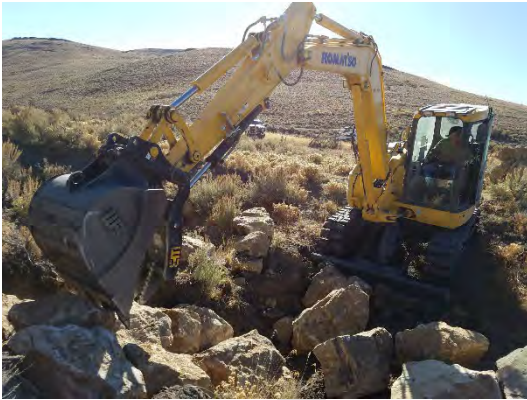
Figure 24. Installing an artificial riffle or low rise in-channel rock structure for grade control (left). Installed low-rise in-channel rock structure (right).
