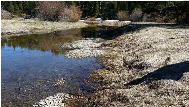
Figure 21. Completed bank revetment with willow staking (left). Completed gully revetment (right). (Image Source: USFS)
