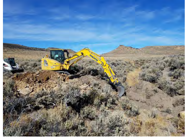
Figure 23. Back-filled headcut (left). Installing a grade control structure to prevent further downcutting (right). (Image Source: USFS)
