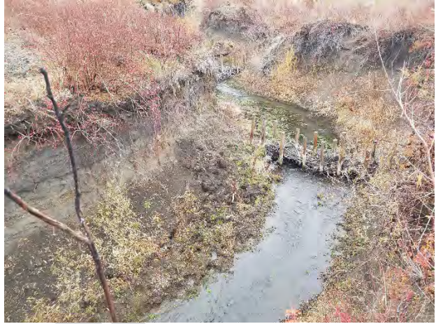
Figure 20. Installation of post-assisted structures (left). Installed in-channel post-assisted structure (right). (Image Source: USFS)
