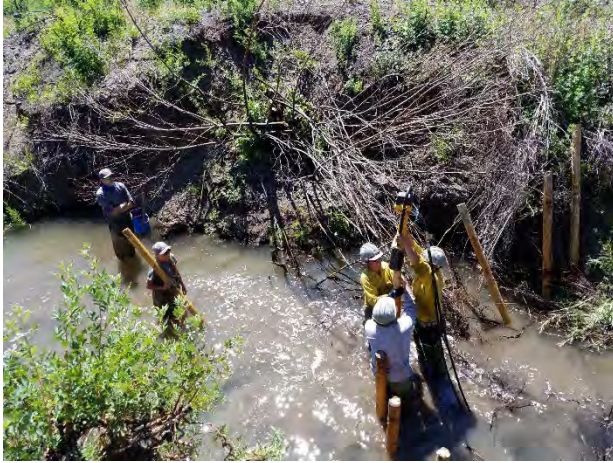
Figure 20. Installation of post-assisted structures (left). Installed in-channel post-assisted structure (right). (Image Source: USFS)
