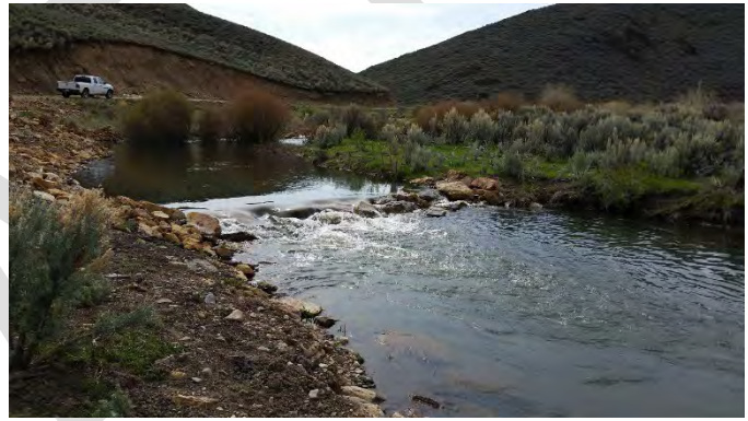
Figure 24. Installing an artificial riffle or low rise in-channel rock structure for grade control (left). Installed low-rise in-channel rock structure (right).
