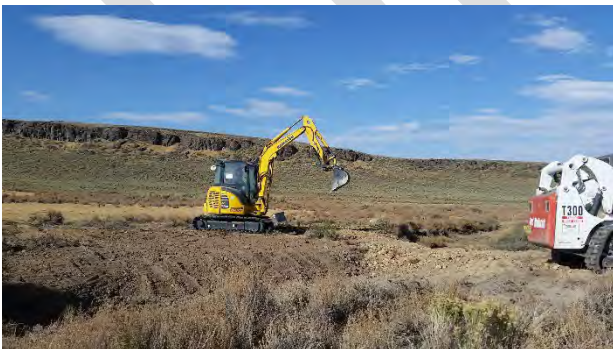
Figure 22. Installation work for a meadow plug and pond feature (left). Completed plug and pond feature in an ephemeral drainage (right). (Image Source: USFS)
