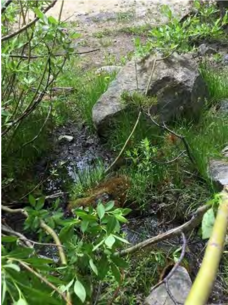
Small pool at base of collapsed adit
