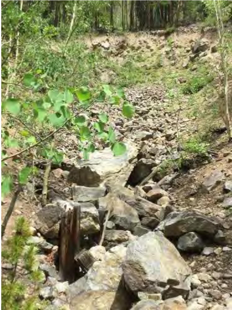
Bard Creek Mine - Reliance Mine: Collapsed adit next to pile
