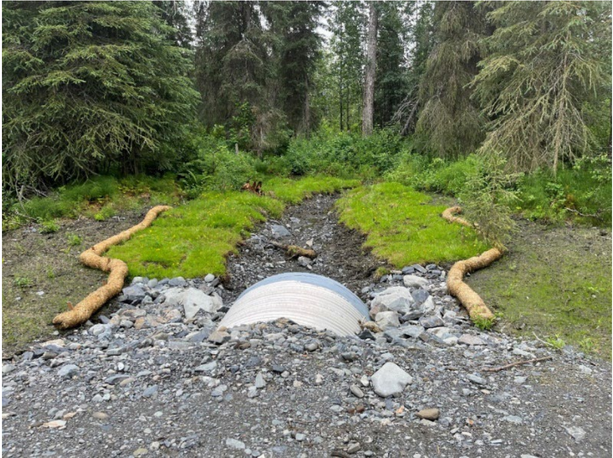
Figure 4. The Center TS Road culvert replaced by ADOT in 2024.
