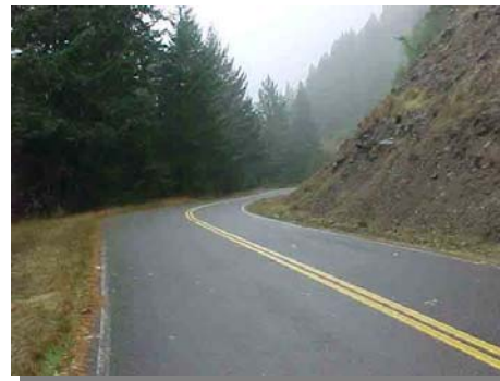
Stabilized mid-slope road
