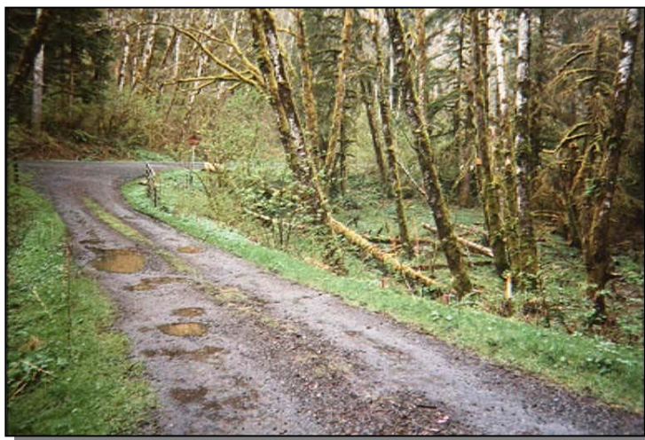
Typical "High clearance" Key Forest road
