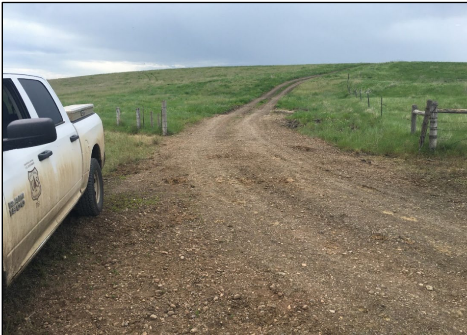
Figure 39. Stable geotextile fabrics two years after installation. Forest Service Road #203, Fort Pierre Geographic Area. Photo June 2021 by Dan Svingen.
