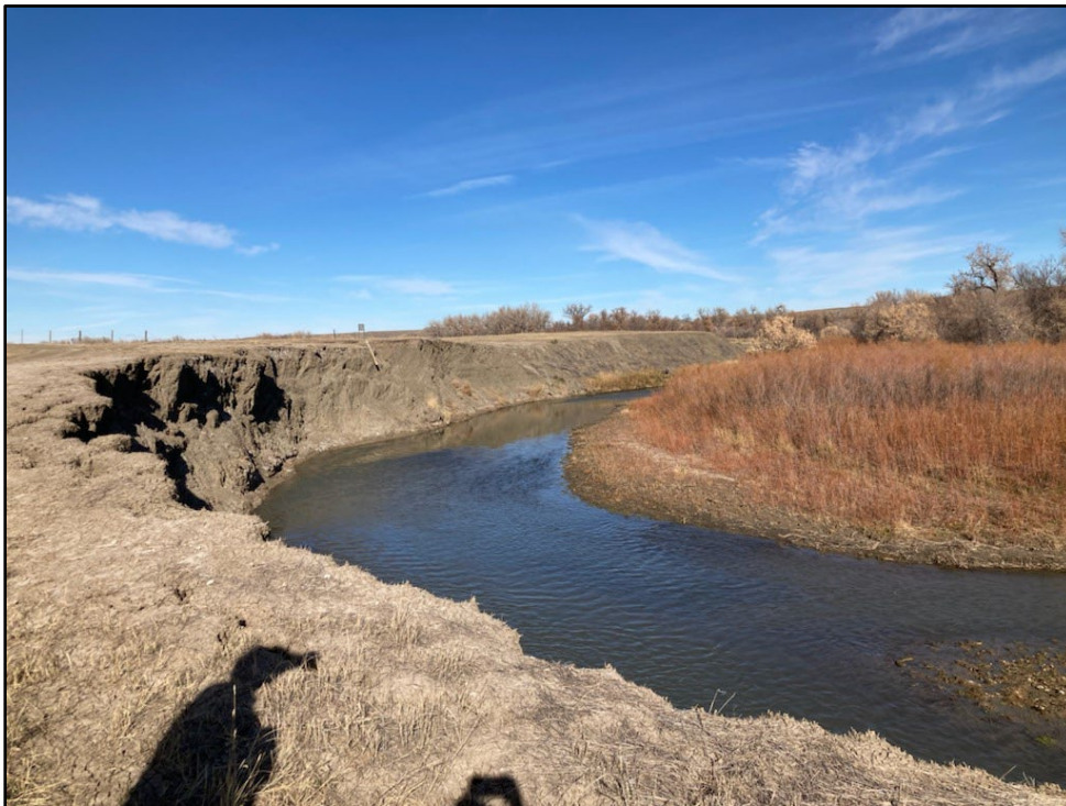
Figure 6. Rapid Creek in Cole Draw Allotment at site of old railroad bridge, looking upstream. Note eroding bank. Photo November 2021 by Julie Wheeler.
