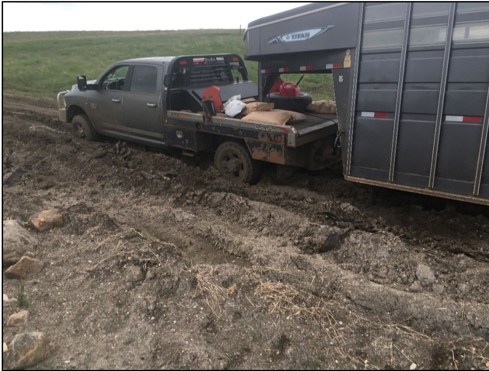
Figure 40. Vehicle high-centered atop failed geotextile fabrics. Forest Service Road #253, Fort Pierre Geographic Area. Photo May 2020 by Dan Svingen.
