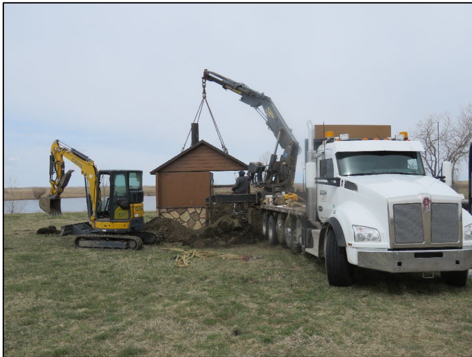
Figure 27. Installing a sweet-smelling toilet (SST) at Richland Dam Dispersed Recreation Area, Fort Pierre Geographic Area. Photo April 2020 by Dan Svingen.
