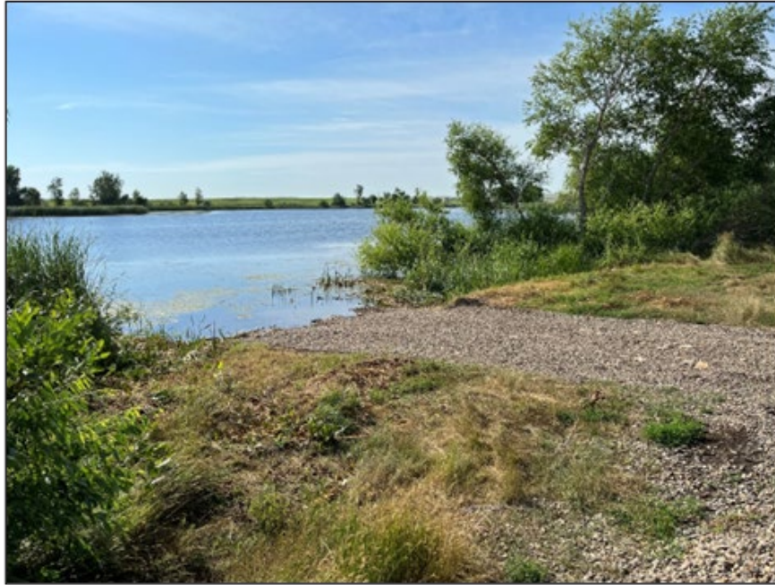
Photo: 2. Newly installed, graveled boat ramp at Sheriff Dam. July 2023.
