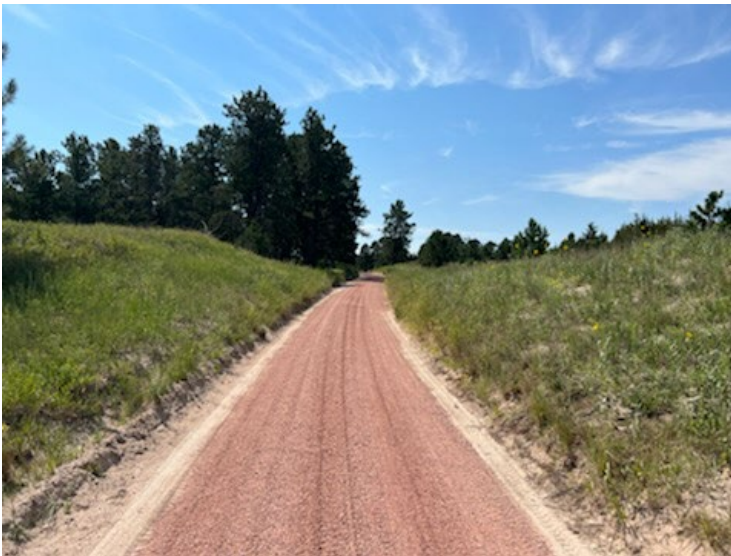
Photo: 9. FR 203 After GAOA. Gravel aggregate placed to fortify road surface.
