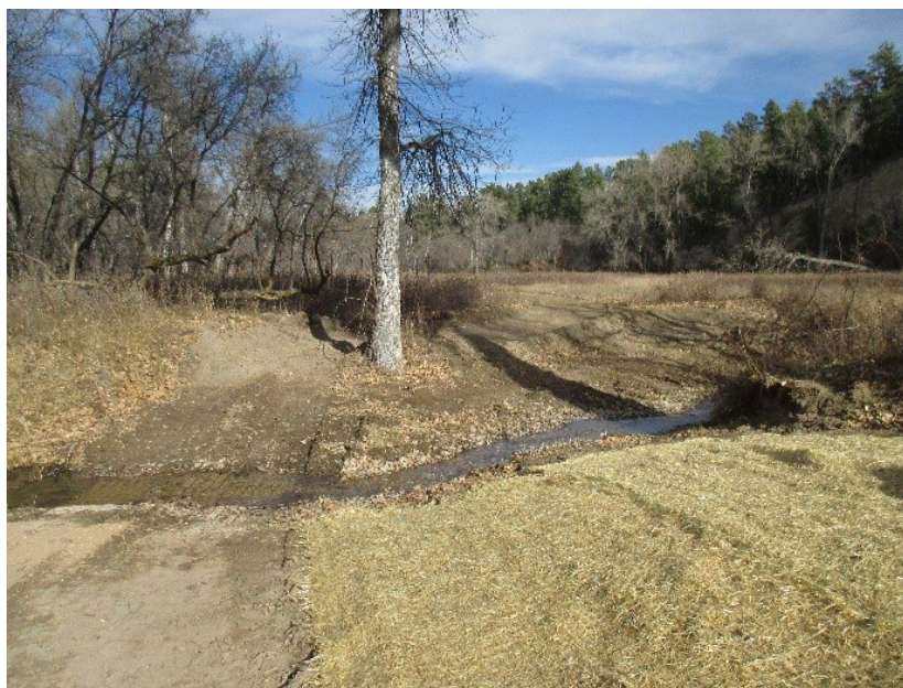
Photo: 14. After: stream is restored to its natural channel and a hard crossing prevents sedimentation from vehicles.
