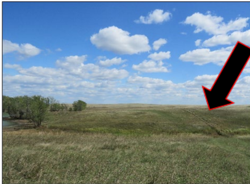
Photo: 3. Old location of Forest Service Road 219-A, looking east. Note rutted crossing of swale (arrow). September 2017.
