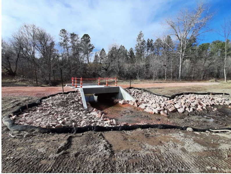
Photo: 12. After: Improved culvert structure with simulated streambed for aquatic organism passage and increased flood resiliency.
