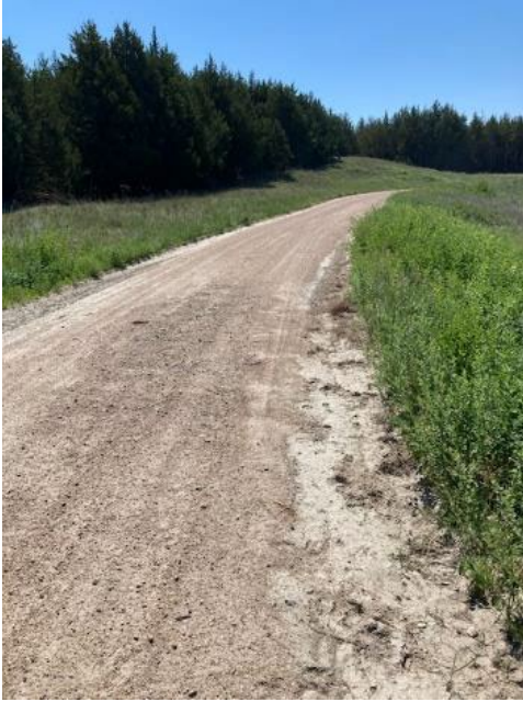
Photo: 8. FR 203 before GAOA. Road improved with clay base funded by Nebraska Recreational Trails Program.
