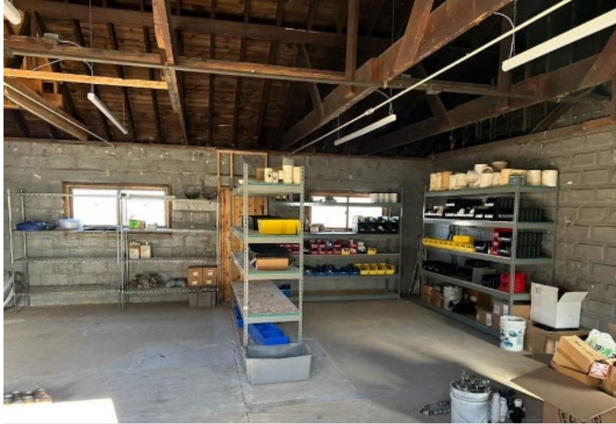
Photo: 10. View of the Nursery shop after the demolition of the inside. The space is now being used to store items needed in the day-to-day running of the nursery including wood, irrigation supplies, and more.
