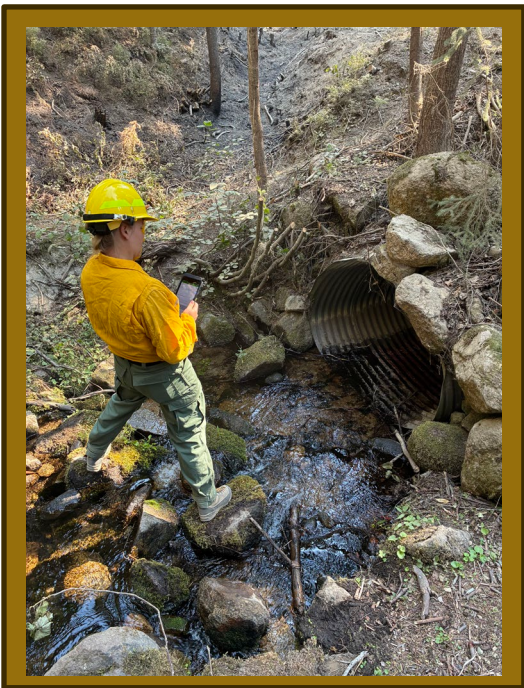
Figure 3. Engineering specialist assessing road infrastructure on the Anthony Fire.
