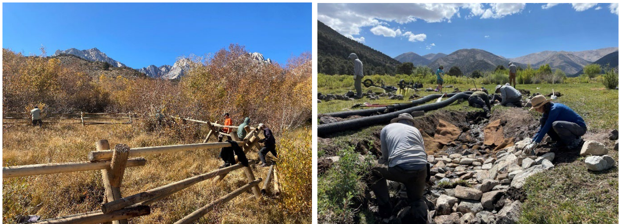
Figure 10: Installation of buck and rail fence around sensitive fen in Birch Creek Meadow (left) and construction of Zeedyk restoration structure in Davis Creek Meadow (right)
