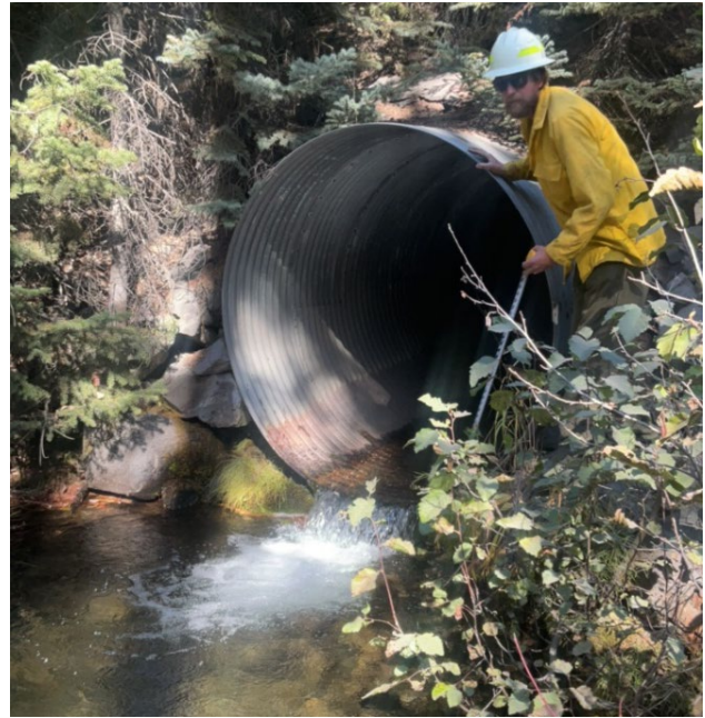
Figure 3. Fisheries specialist surveying a culvert near the McCully burned area.
