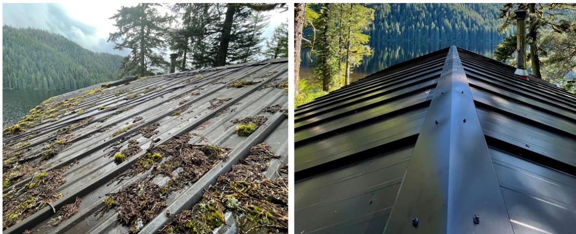
Before and after view of the Southeast Heckman cabin roof.
