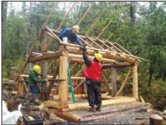
The Three Lakes Shelter is rebuilt using both old and new components.
