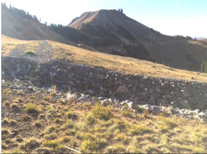
PHOTOGRAPH 1 View of rock ditch and established vegetation, facing
