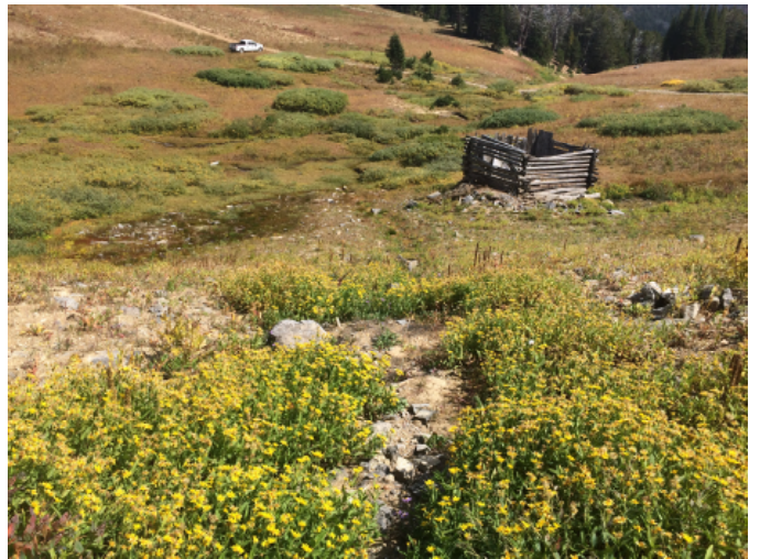
PHOTOGRAPH 4 View of drainage ditch facing east
