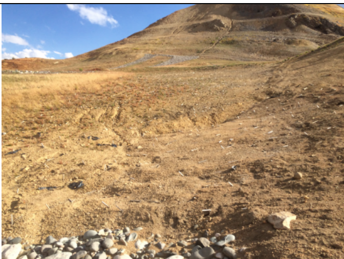
PHOTOGRAPH 5 View of erosion occurring in bare soil area, facing south
