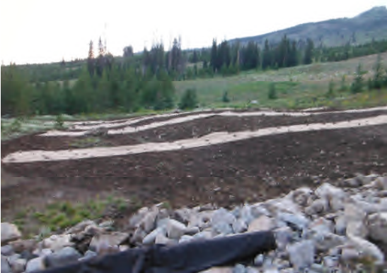
Erosion mat on gallery.
