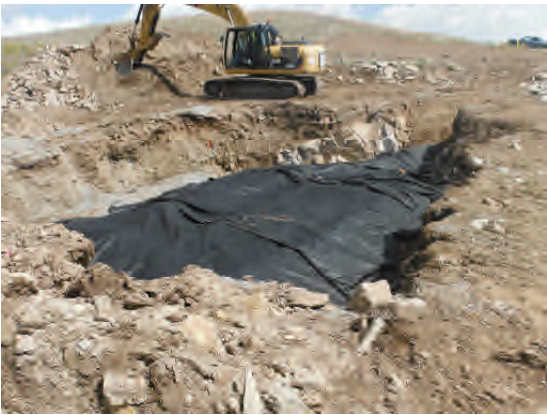
Geotextile in place over gravel fill.
