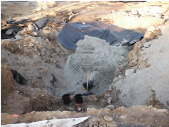
Partially backfilled sump liner patch.
