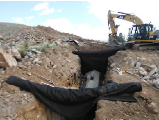
Drainpipe being wrapped with geotextile.
