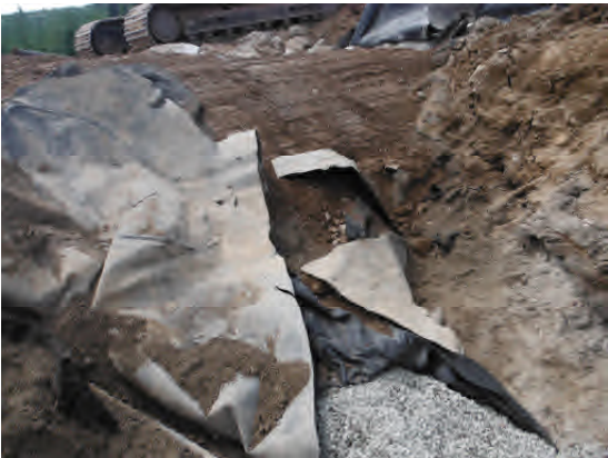
Replacing original sump bottom liner.
