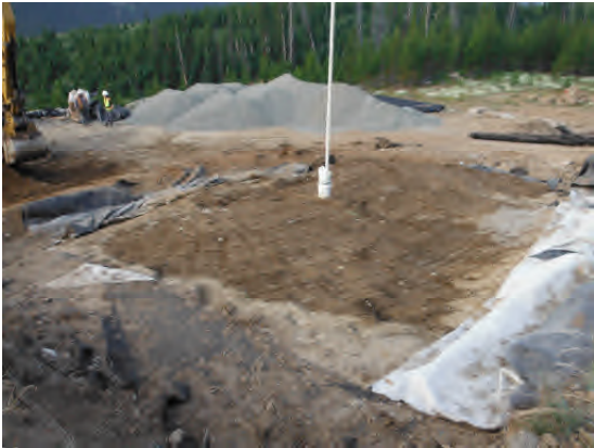
Compacted waste prior to liner replacement.
