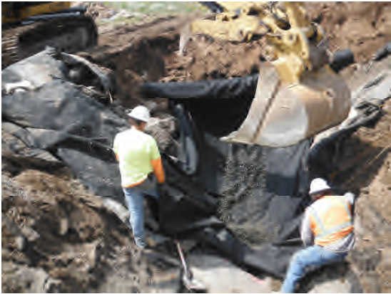
Placing bedding gravel and geotextile into drain pipe trench.
