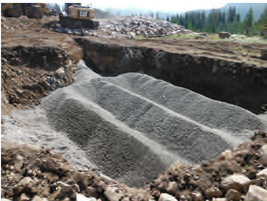
Gallery being backfilled.
