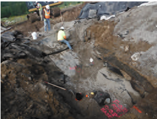
Cutting into sloped portion of bottom liner.
