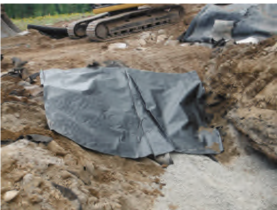
LDPE patch in place over sump liner prior to backfilling.
