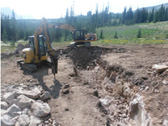
Trench and infiltration gallery excavation at end of day.
