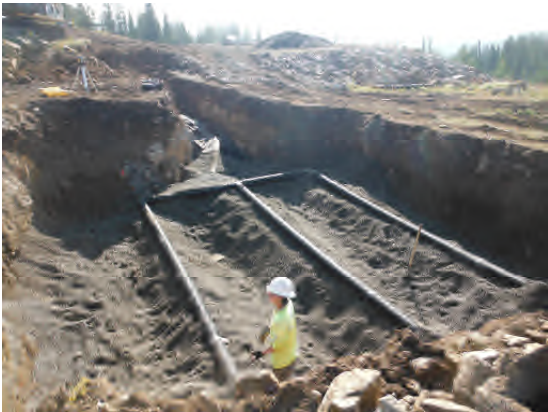
Middle lateral pipe is installed and surveyed.
