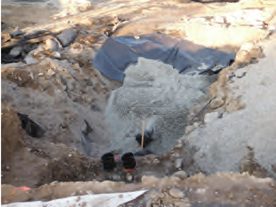
Partially backfilled sump liner patch.
