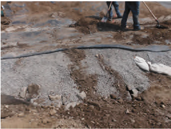
Anchor trench along western edge of repository.
