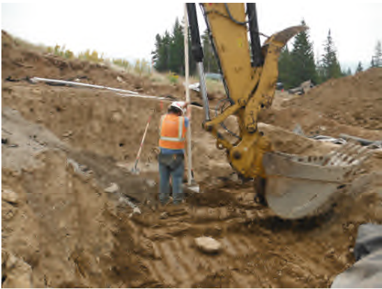
Placing non-slotted portion of sump access tube.
