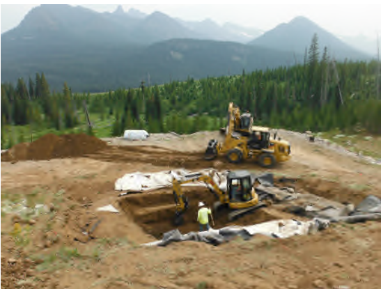
Waste excavation and stockpiling.
