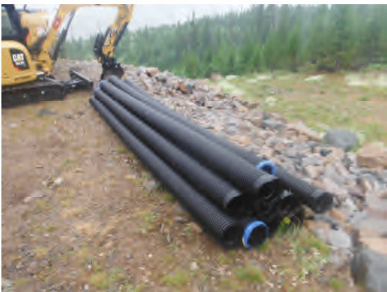
Slotted and solid (marked with blue) HDPE drain pipe.
