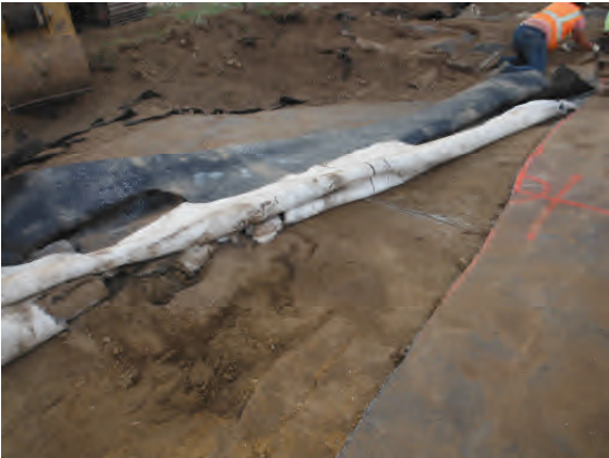
Close up of waste beneath cut liner.
