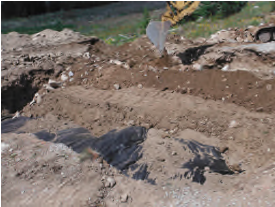
Cover soil being backfilled into gallery.
