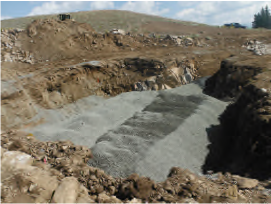
Completed gallery gravel backfill.
