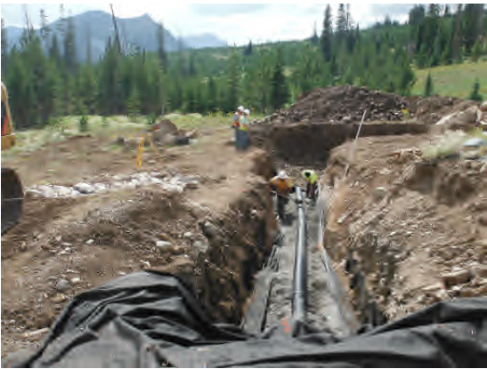
Installing drain line into gallery.
