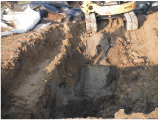
Filtration layer sand in excavated trench.
