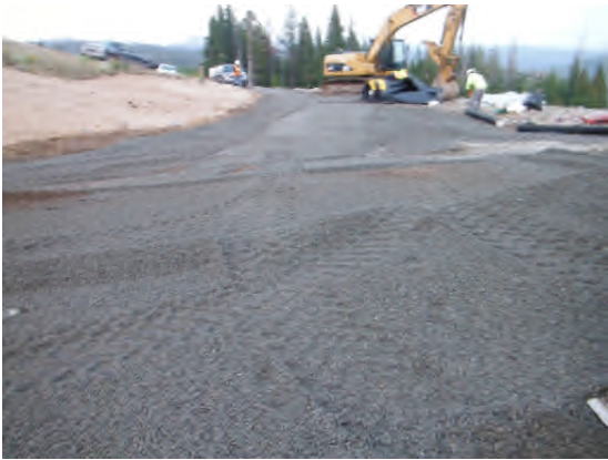
Spreading gravel on access road.
