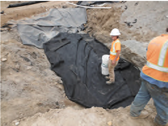
Placing geotextile above sump gravel.
