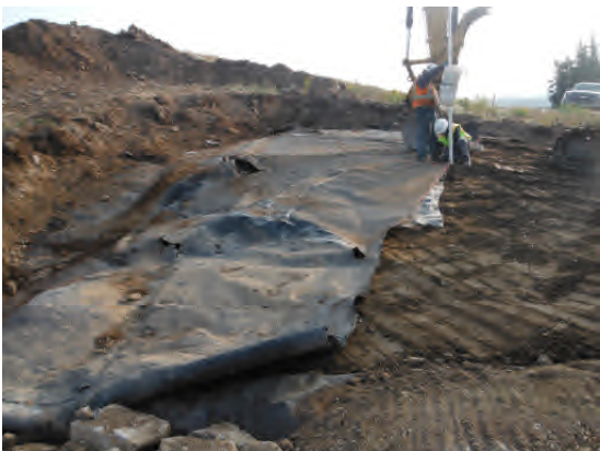
Replacing north/uphill side of original liner.
