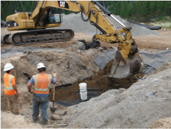
Placing waste material above geotextile.
