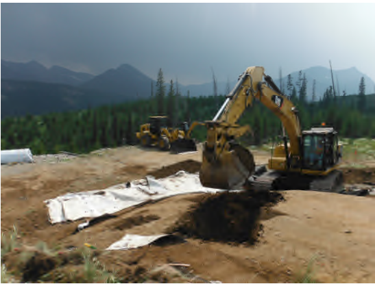
Beginning to excavate mine waste from repository.
