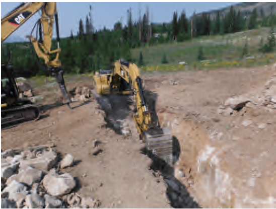
Excavating drain pipe trench.
