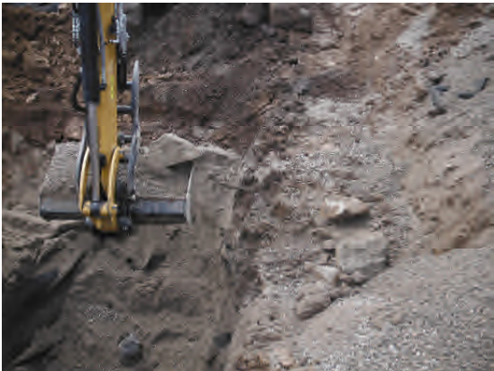
Close up of rocks found in gravel drainage layer.
