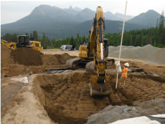
Compacting backfilled waste.
