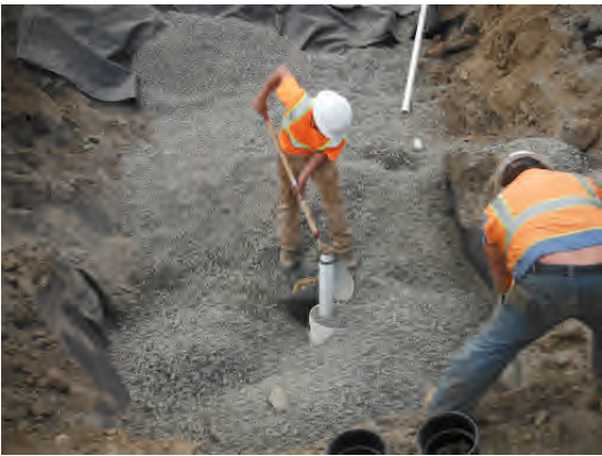
Levelling sump gravel backfill.
