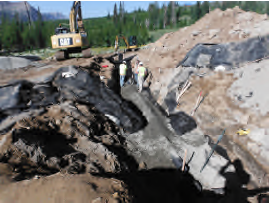
Surveying elevation of drain pipe to ensure correct grade.
