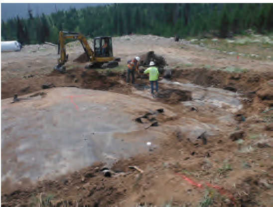
Wide view of exposed cover liner.
