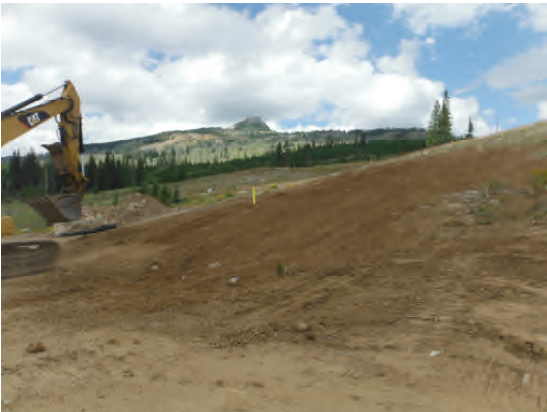
Final cover soil replacement.
