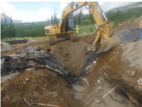
Excavating trench westward from sliced liner.
