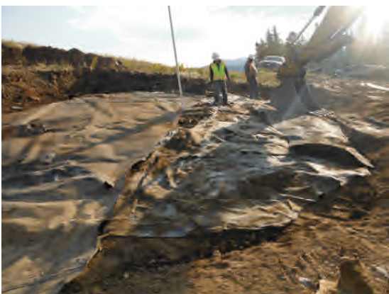
Replacing downhill side of GCL.
