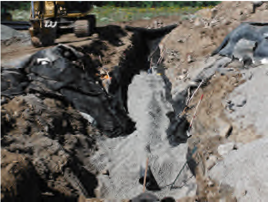
Backfilling drain pipe / trench.
