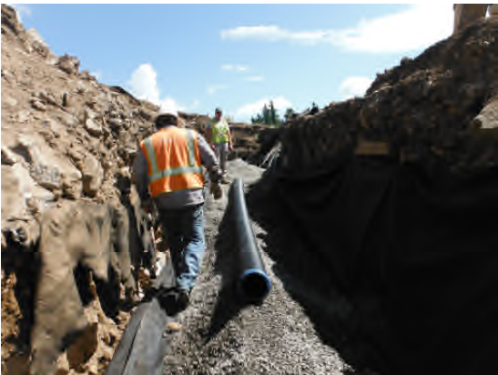
Placing another length of pipe.
