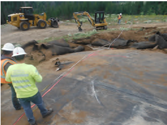
Marking center line for cutting liner.
