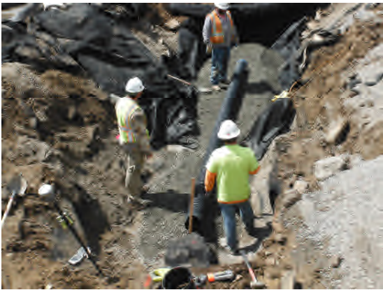
First section of drain pipe in trench/sump.
