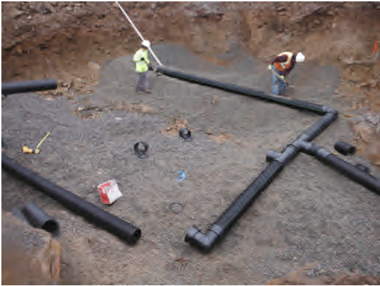
Infiltration pipe installation in progress.
