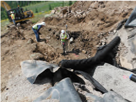
Surveying trench through access road.
