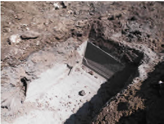
Close-up of sand layer (appx 20" thickness of sand).
