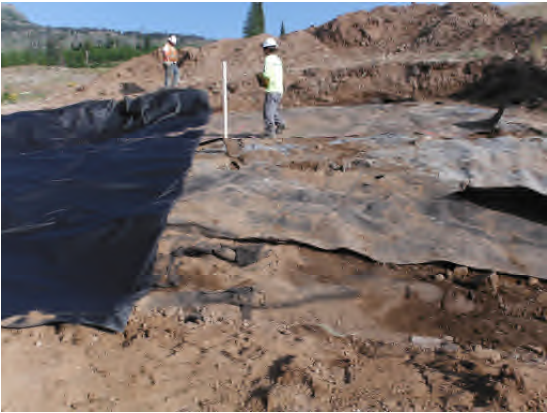
Pulling LDPE patch into place.
