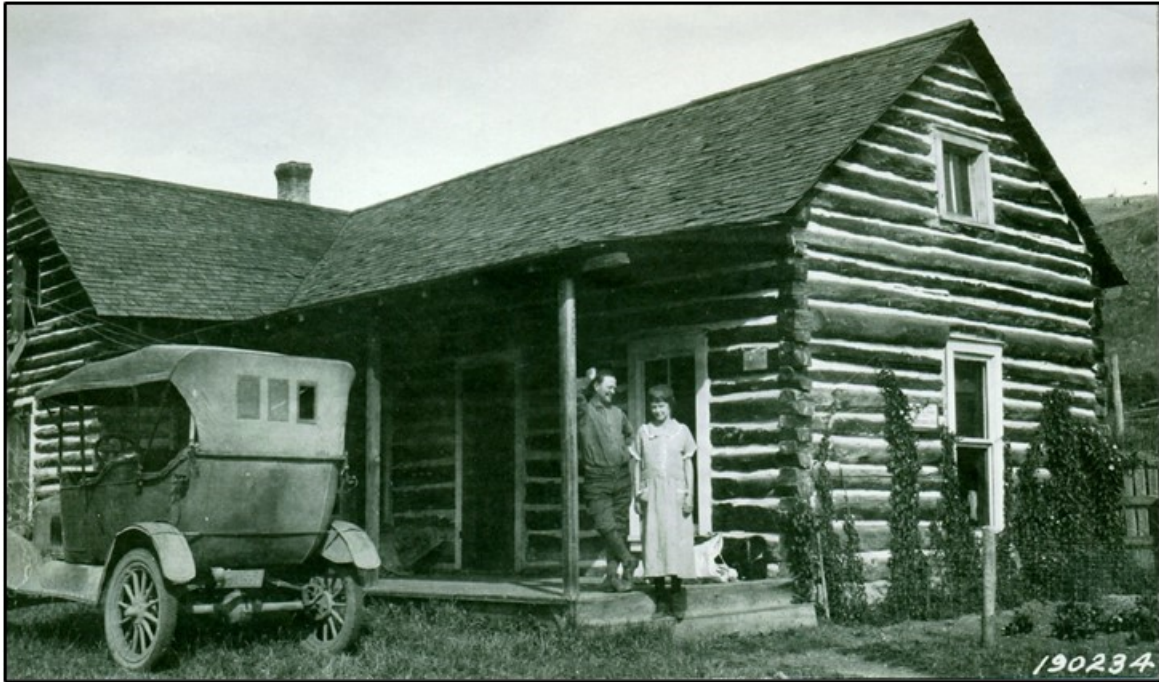
MT_StillwaterCounty_MeyersCreekWorkCenter_0002. Meyers Creek Ranger Station with addition in 1924, looking northwest. (Photographer: M.H. Wolff; Custer Gallatin National Forest Photo GNF190234)
