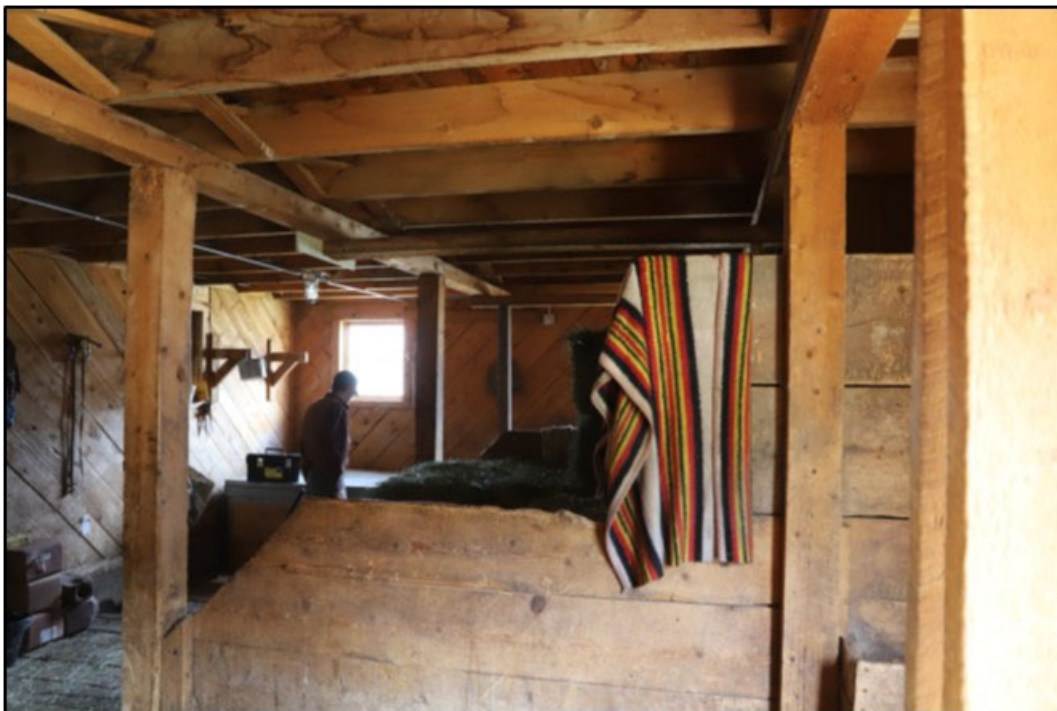
MT_StillwaterCounty_MeyersCreekWorkCenter_0021. Interior view of the Feature 4 barn tack room, May 19, 2022, View to east. (Photographer: Tim Urbaniak)
