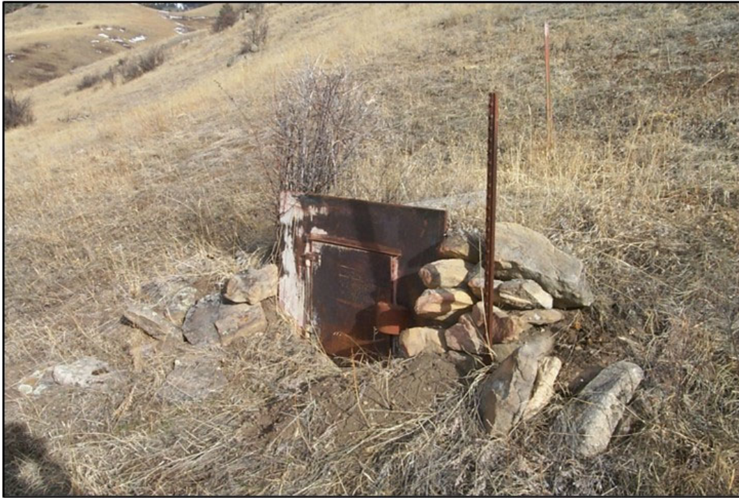
MT_StillwaterCounty_MeyersCreekWorkCenter_0030. The Feature 15 explosives storage structure, March 27, 2002, View to west. (Photographer Mike W. Bergstrom)
