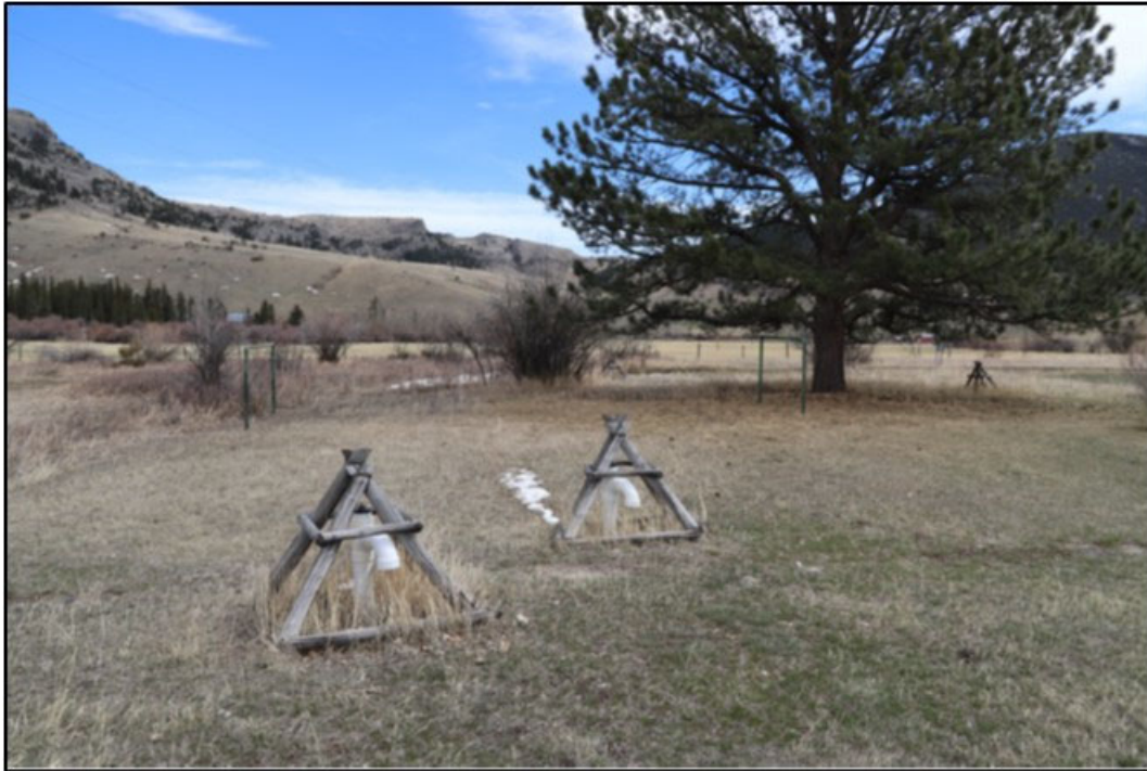
MT_StillwaterCounty_MeyersCreekWorkCenter_0026. View of the protective log buck structures at site water and effluent fixtures, May 19, 2022, View to east. (Photographer: Tim Urbaniak)
