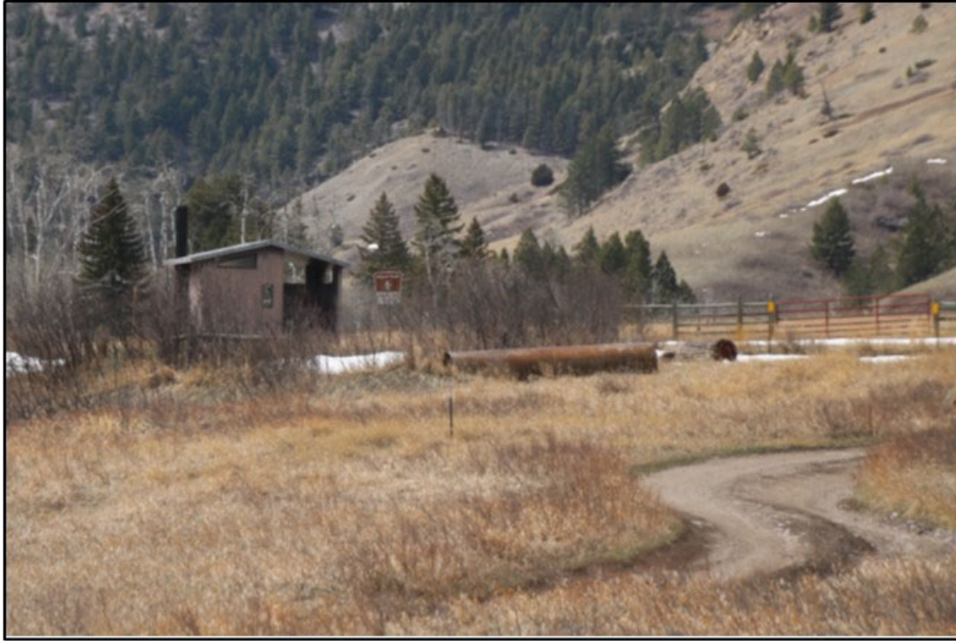
MT_StillwaterCounty_MeyersCreekWorkCenter_0024. View of the noncontributing latrine (Feature 14) at the Meyers Creek Trailhead, May 19, 2022, View to west. (Photographer: James Busse)
