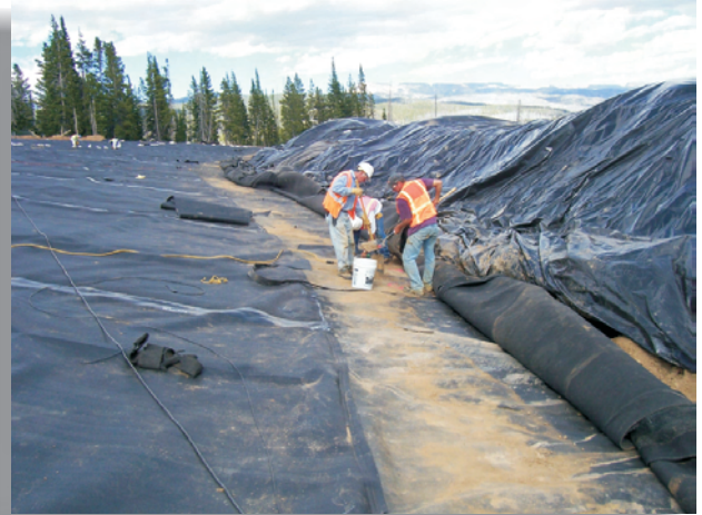
Expanding the New World Waste Repository Bottom Liner - July 2005
