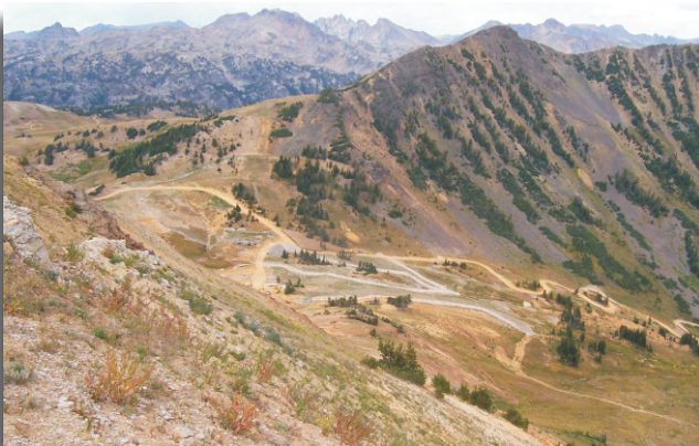
Reclamation Work in the Headwaters of Fisher Creek
