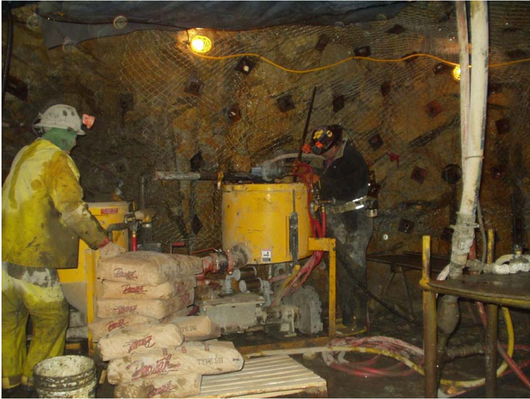
Figure 17. Grouting the 1066 Fault Zone
