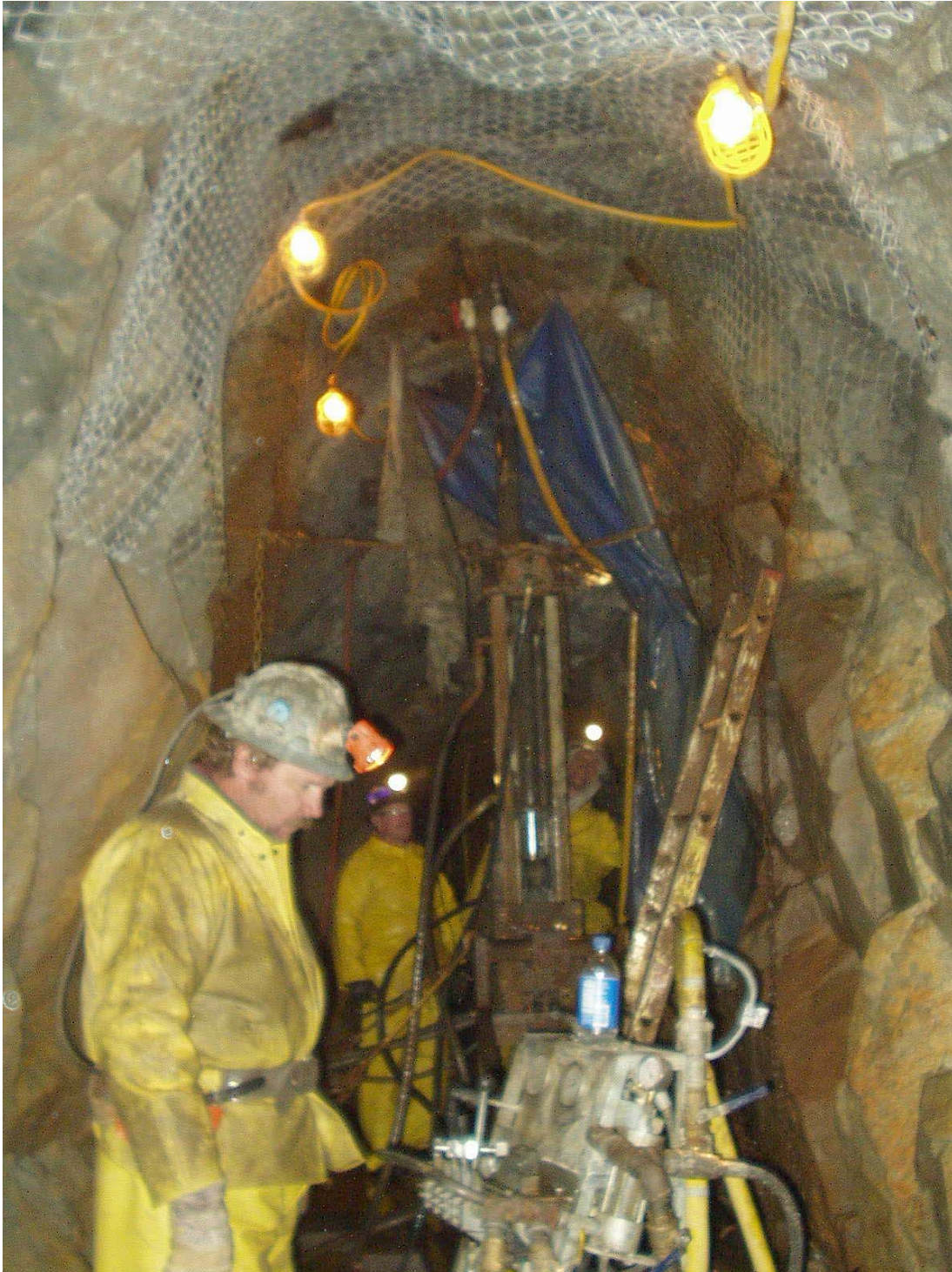
Figure 25. Watertight Plug Station with Hagby Core Drill Drilling Borehole to Surface
