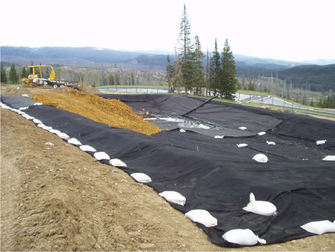
Figure 9. Muck Storage Pad at the New World Waste Repository
