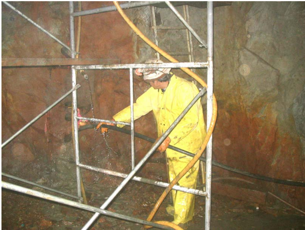
Figure 32. Flushing an Underground Borehole in the Gold Dust Adit
