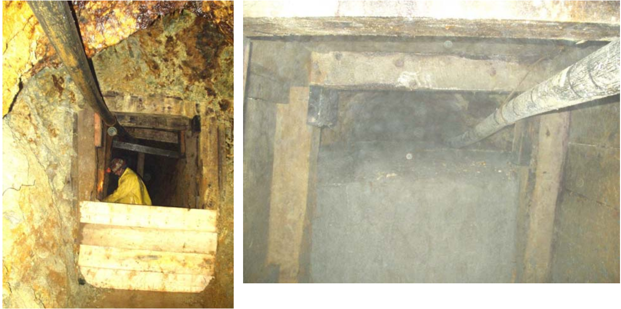
Figure 28. Cement Backfilled Segment
