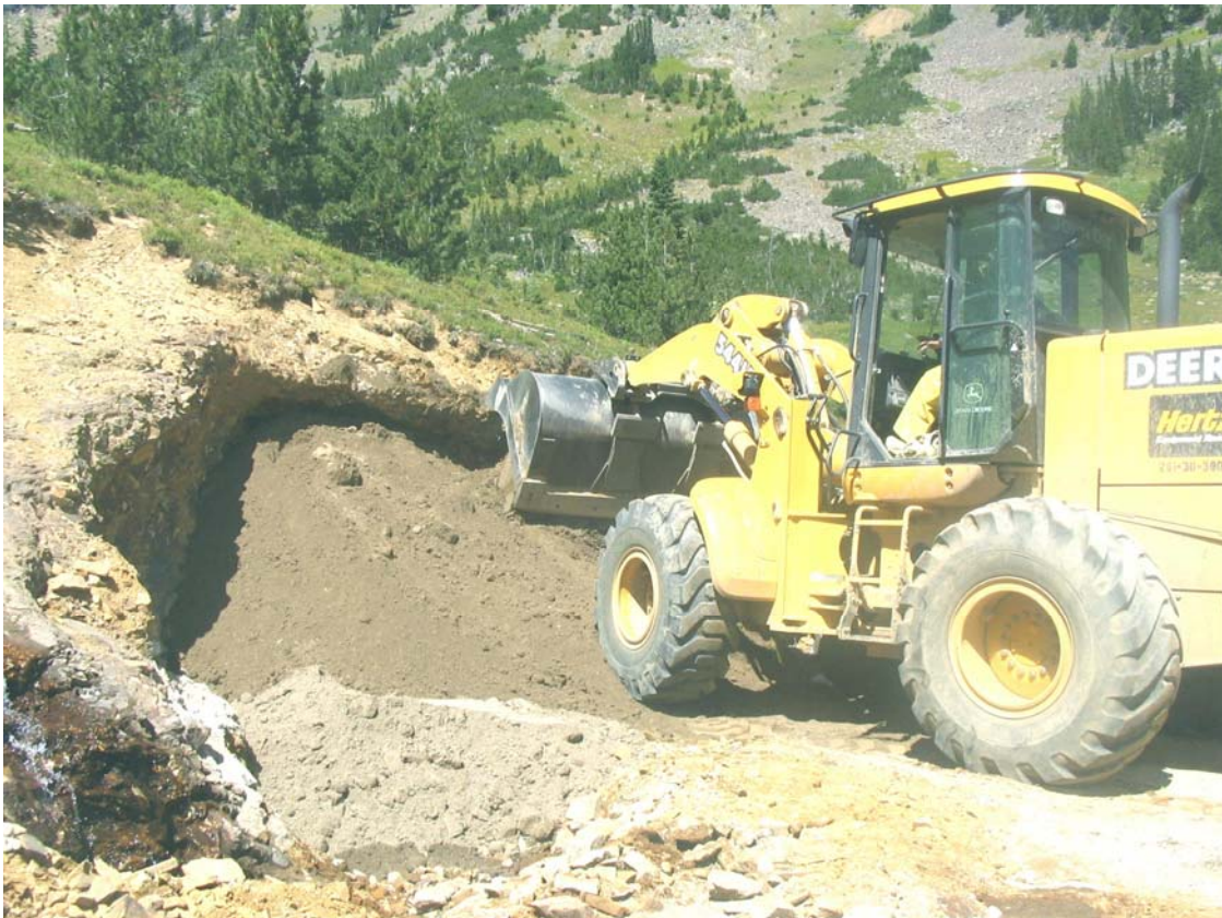
Figure 30. Backfilled Adit Portal Plug
