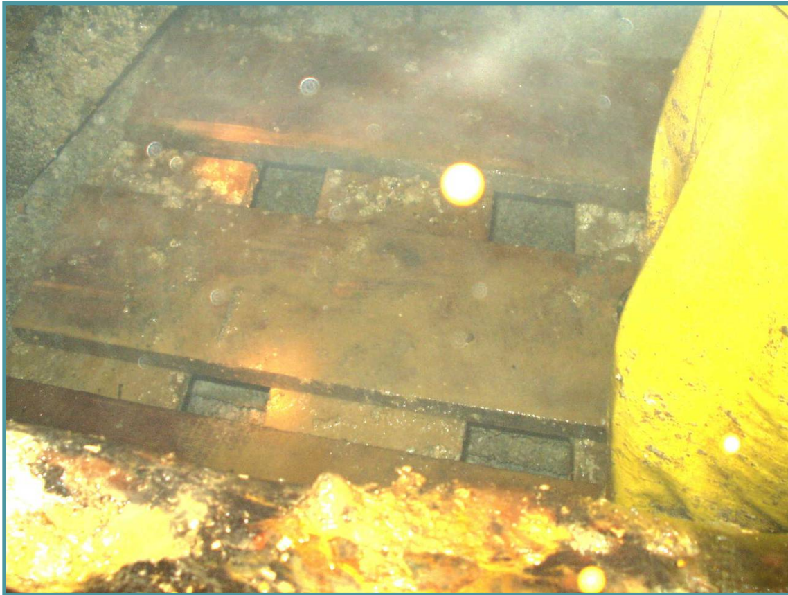
Figure 22. Wooden Lattice Mat Installed Over Bentonite Pellet Clay Layer
