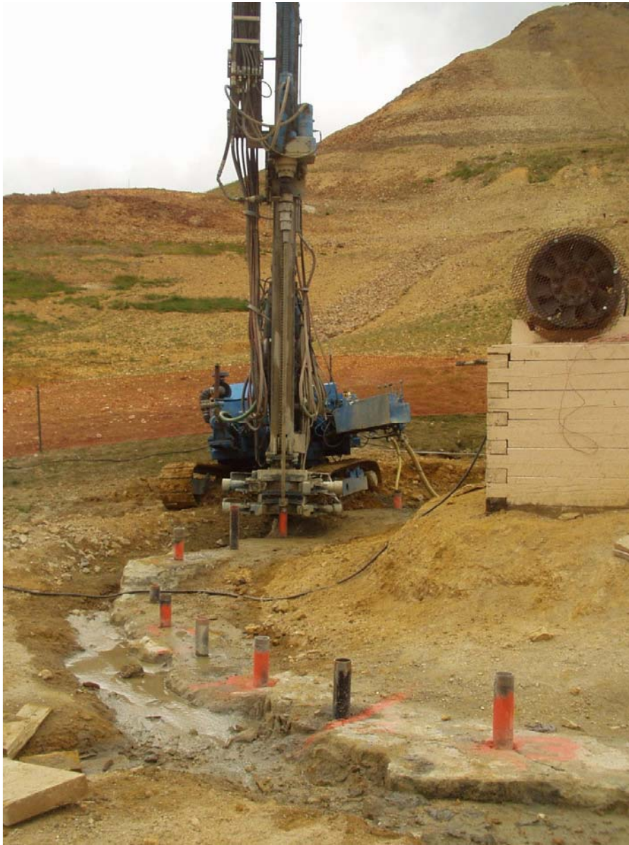
Figure 14. Rotary Drilling Primary (Red) and Secondary Drill Holes into Bedrock
