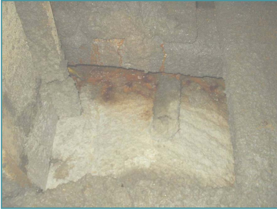
Figure 21. Cement Backfill in Timbered Portion of the Como Raise
