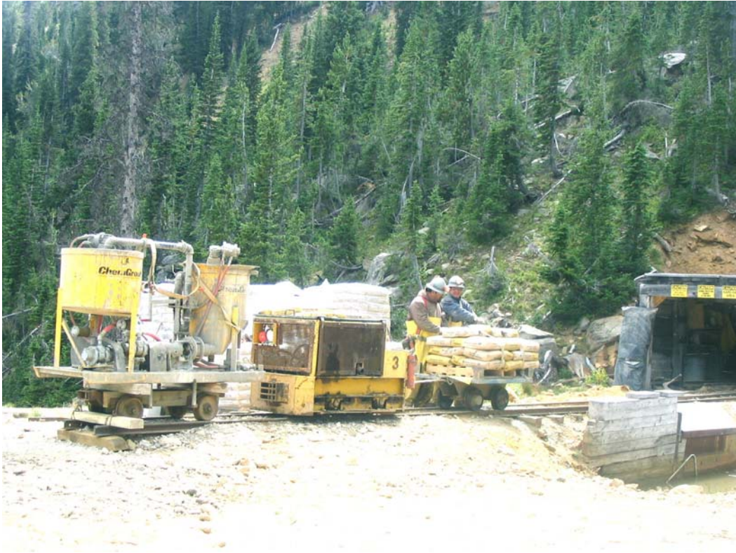
Figure 31. Gold Dust Adit Rehabilitation
