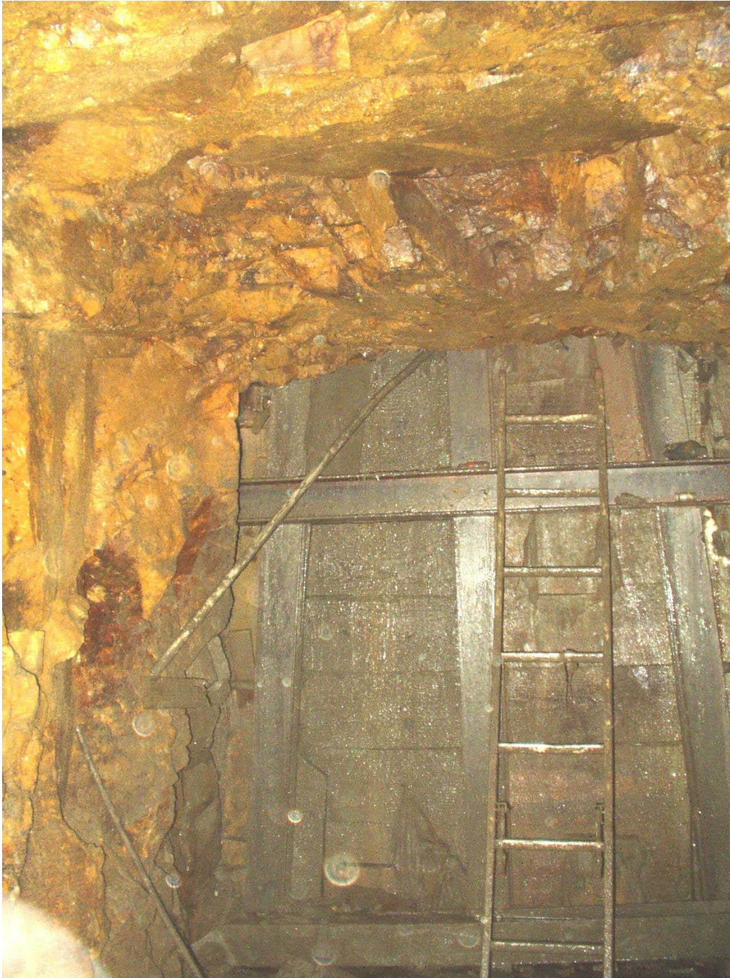
Figure 27. I-beam and Timber Constructed Bulkhead for Plug Station
