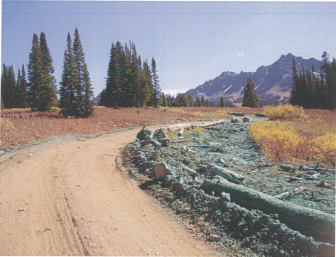
Photograph 10 – Section of Lake Abundance Road Reclaimed to Single Lane
