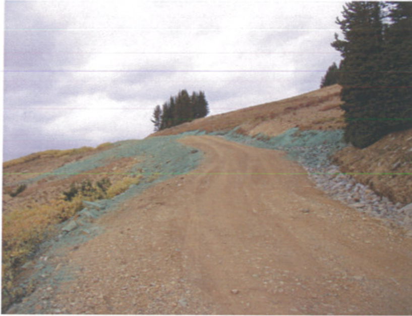
Photograph 11 – Armored Ditch along the Daisy Pass County Road
