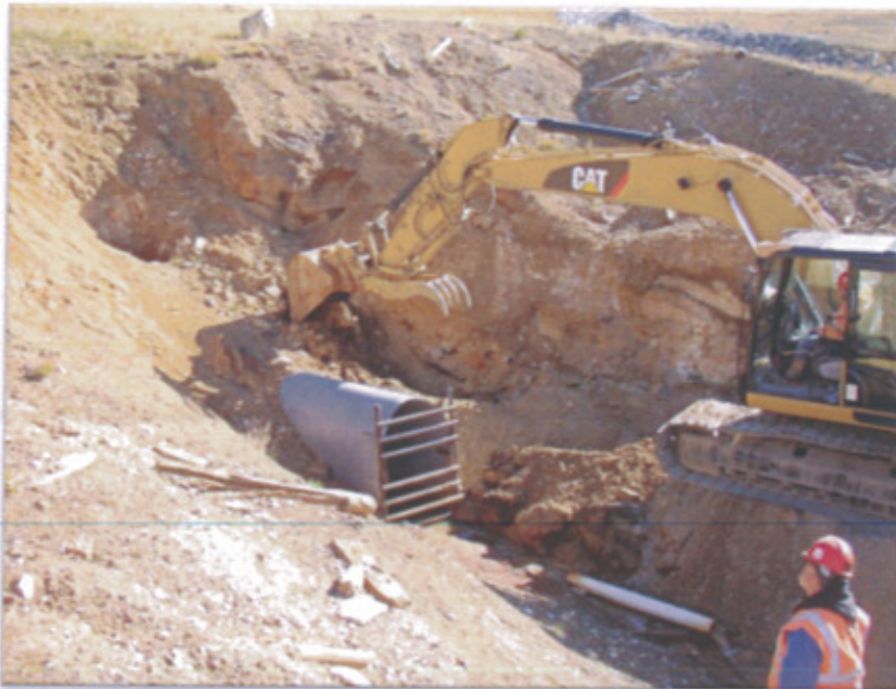
Photograph 1 – Stabilizing McLaren Adit prior to Entry
