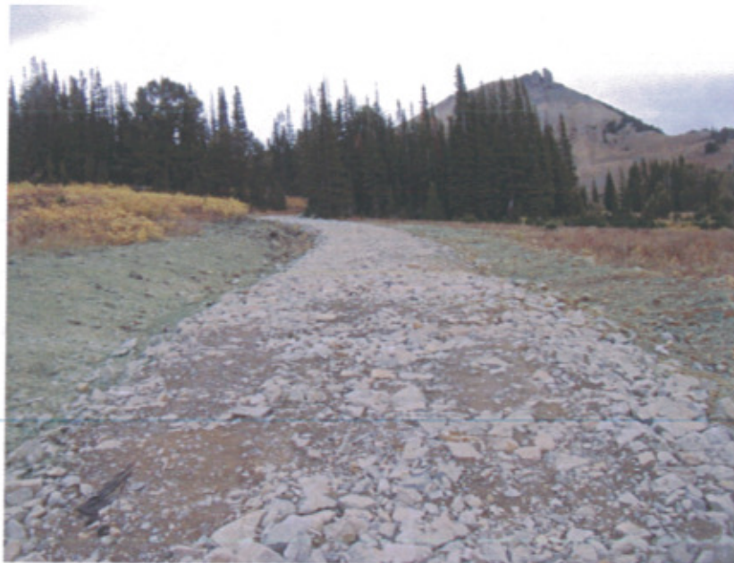
Photograph 9 – Same Section of Road after Stabilization
