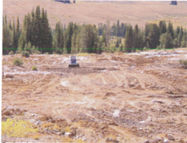
Photograph 18 – Applying Compost below the McLaren Adit
