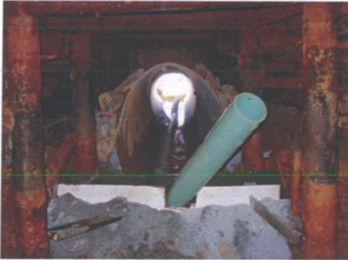
Photograph 2 – Concrete crib wall inside the McLaren Adit
