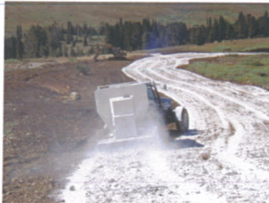
Photograph 17 – Spreading Lime below the McLaren Adit
