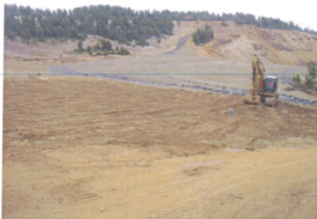
Photograph 6 – McLaren Adit Backfilled and Regraded
