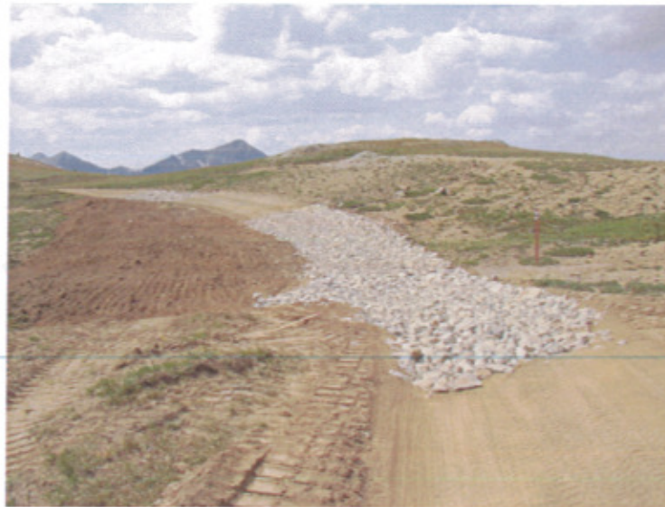
Photograph 12 – Belly Fill along the Scotch Bonnet Road
