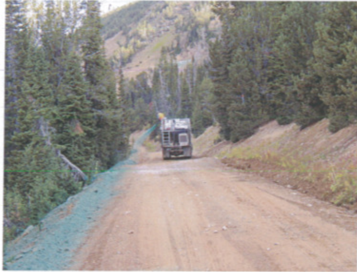
Photograph 20 – Hydroseeding along the Daisy Pass County Road
