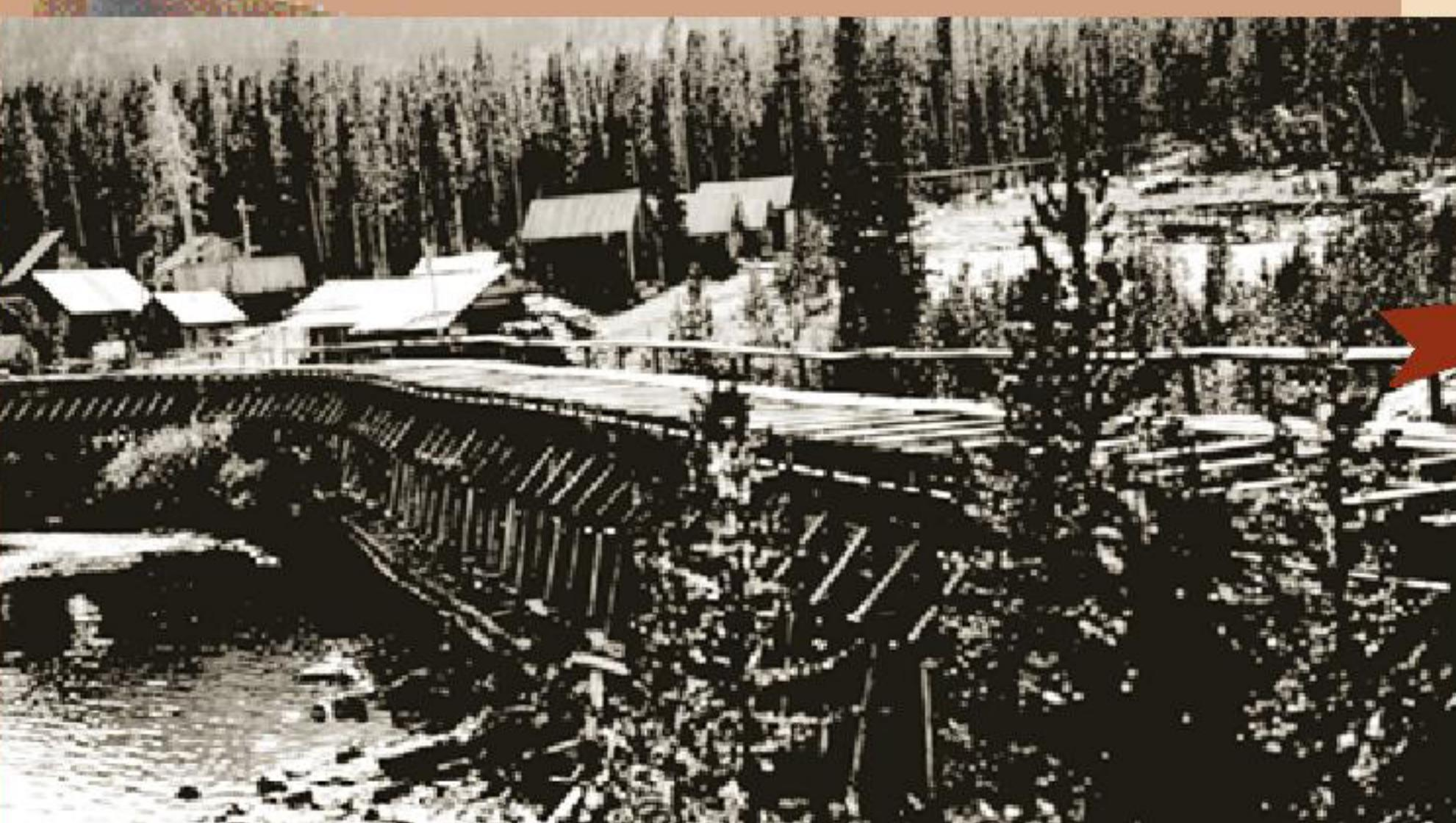
About 80 years ago, a bustling community developed on the site where you are now standing. A power plant was built to supply power to the mining operations on Henderson Mountain. A wooden flume, seen in this photo, carried water to the power plant where the water plunged 50 feet to the powerhouse turbines.
