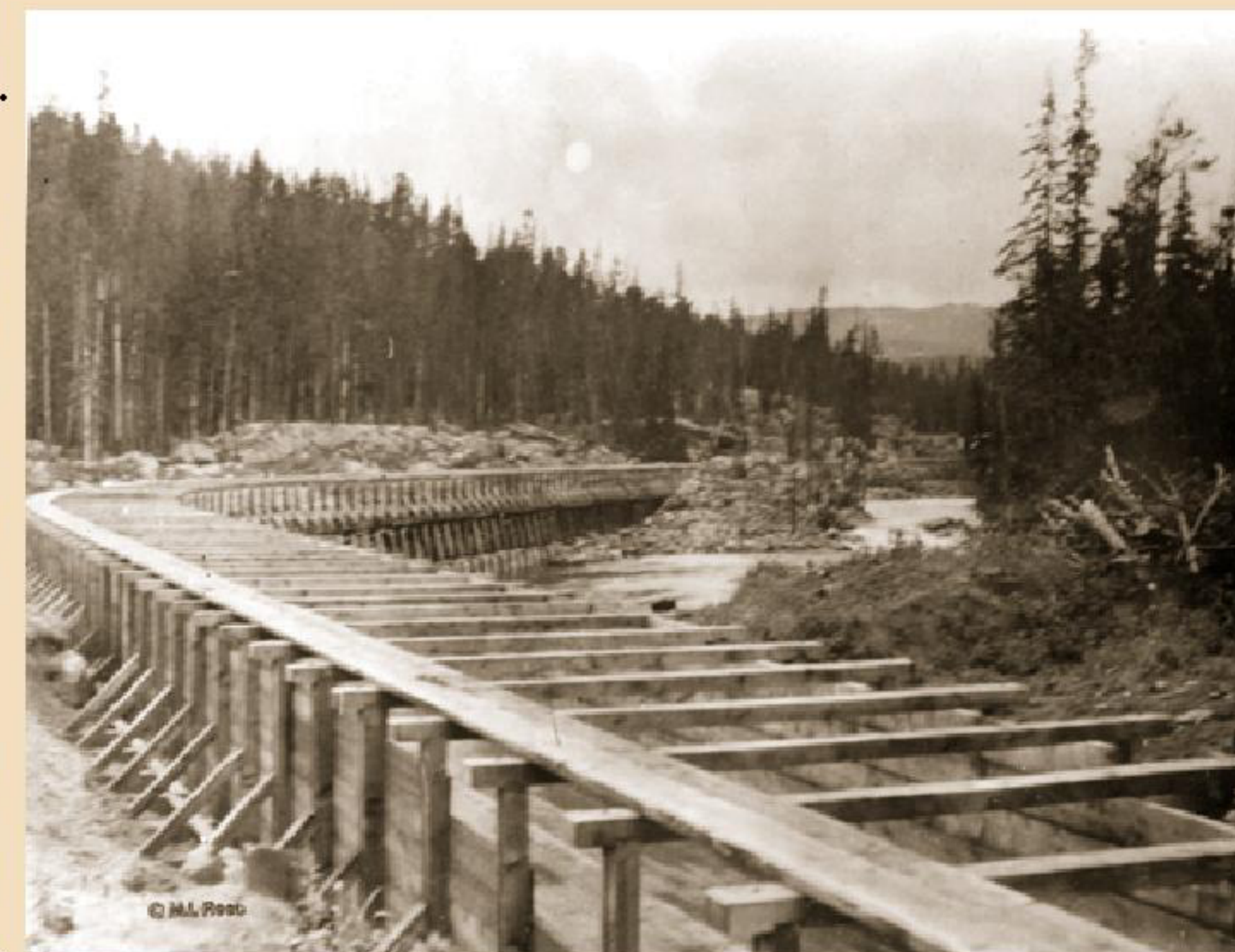
A view to the north of a section of the 1/4-mile wooden flume built to transport water to the Western Smelting and Power Company's Power Plant in 1933.
