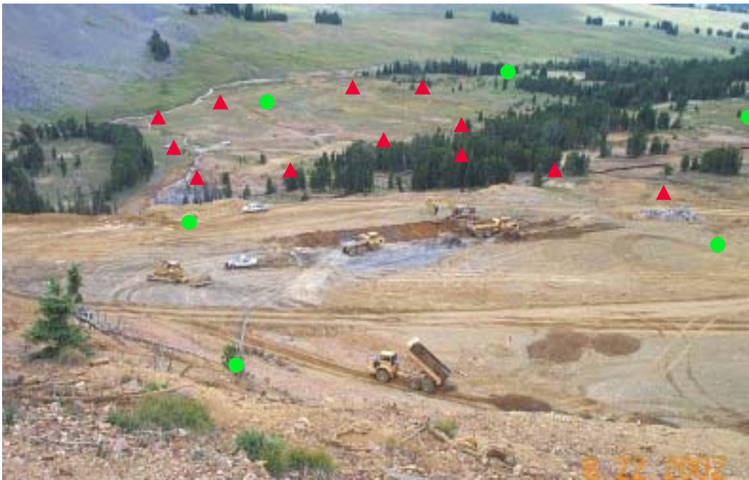
Figure 3. Photograph looking west towards Daisy Creek from the McLaren Pit high-wall showing location of McLaren Pit area piezometers (red triangles) and monitoring wells (green circles).
