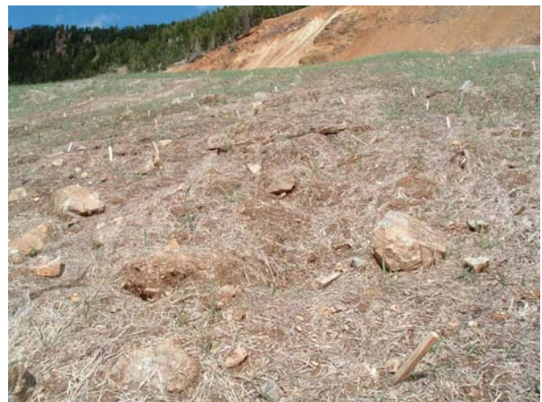
McLaren Pit Cover – Soil Slump on Bench #5 2004 Reclamation Monitoring
