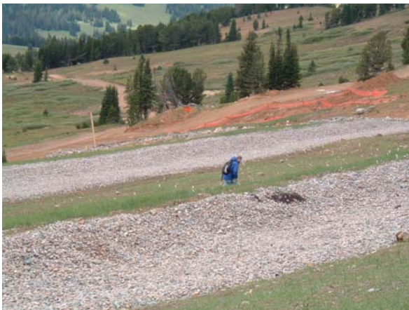
McLaren Pit Cover – Looking SW from Bench #1 2004 Reclamation Monitoring
