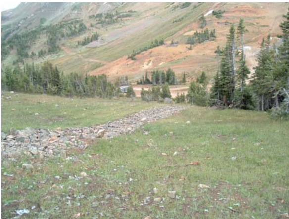
Reclaimed Lower Spalding Dump – August 26, 2004 2004 Reclamation Monitoring
