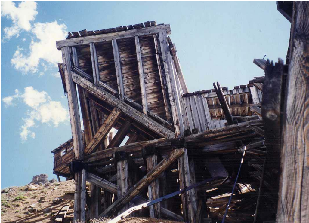
Figure 3-9. Feature 3, upper tram loading terminal, viewing north. Ore bin to left, operator's room in center.
