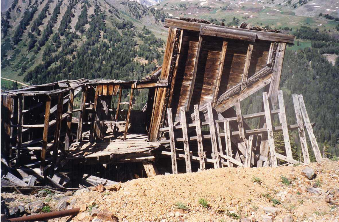
Figure 3-8. Feature 3, upper tram loading terminal, viewing north. Ore bin to right, operator's room in center, bull wheel structure to left. The collapsed loading deck is seen leaning against the ore bin.
