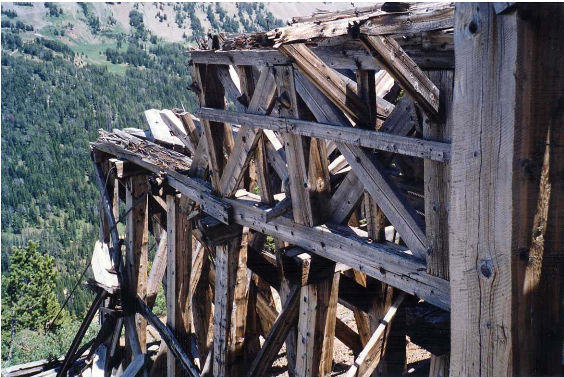
Figure 3-11. Feature 3, upper tram loading terminal, viewing northeast. Bull wheel support structure.
