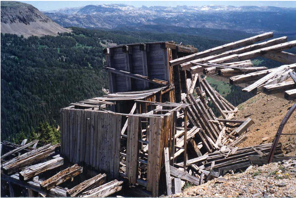
Figure 3-10. Feature 3, upper tram loading terminal, viewing east. Operator's room in center. Portion of Feature 4, trestle in upper right foreground.
