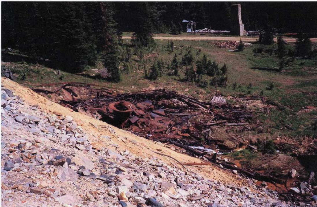
Figure 2-7. Collapsed discharge terminal for the aerial tramway from the Homestake Mine. The Gyratory Crusher is visible in the debris. The long pieces of metal are tram cable guides. The chimney at Feature 13a is seen in the background.
