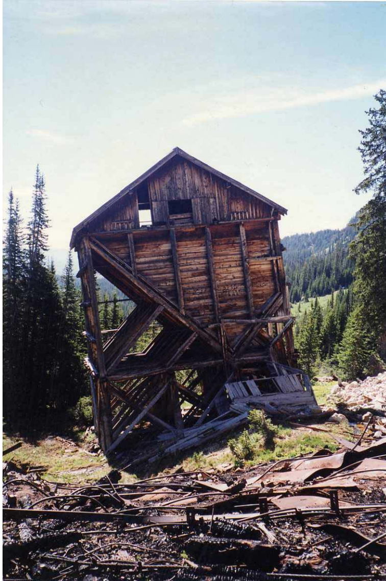
Figure 2-9. Feature 6, ore bin and loading terminal for the lower tramway segment (2001 photo). The remains of Feature 5, the discharge terminal for the upper tram, are in the foreground (note tram cables and cable guides amid the debris).
