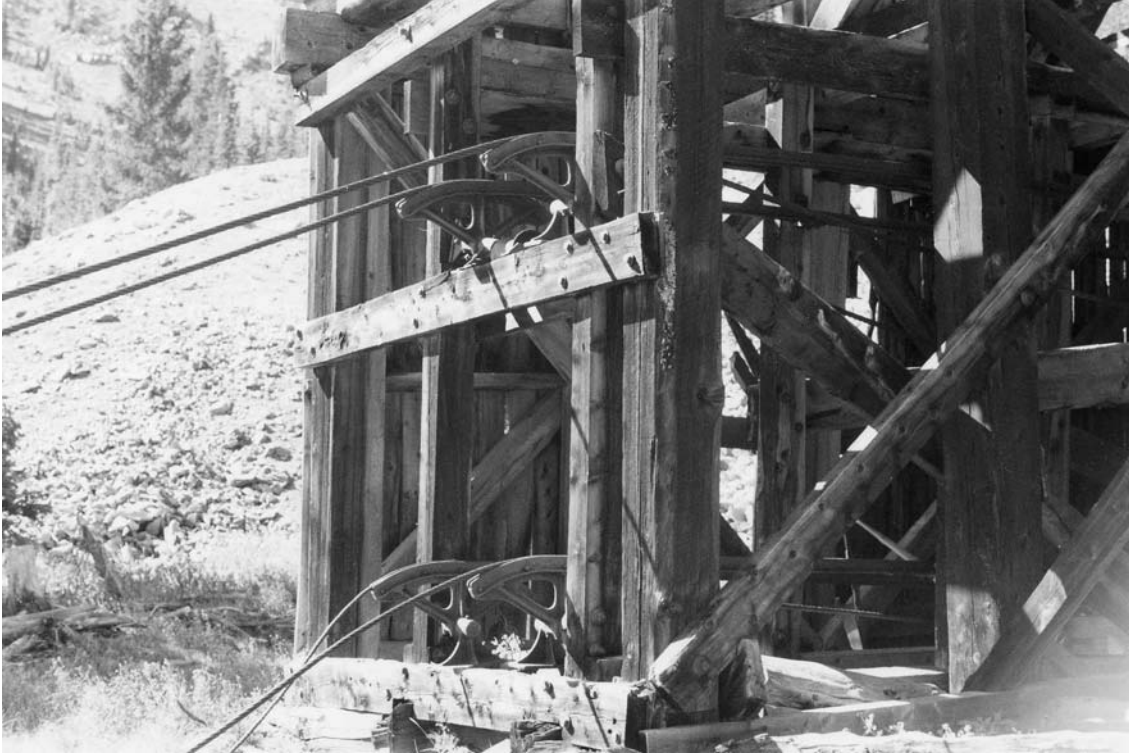
Figure 2-10. Feature 6, Gold Dust ore bin and loading terminal for the lower tramway segment (GCM 1990 file photo). This is the east side of the structure showing the Lawson style terminal where empty cars arrived upside-down on the bottom stationary cable-track, invert and are loaded, then proceed down the line to the smelter.
