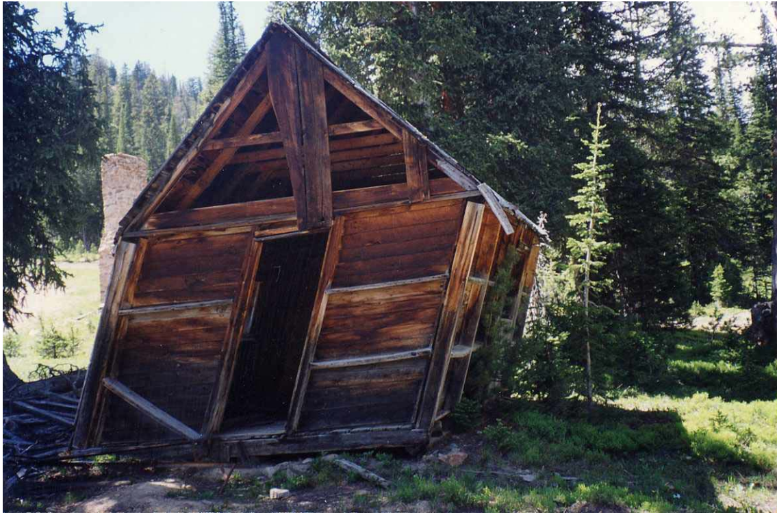
Figure 2-11. Feature 8. One of the few standing structures remaining at the site, this cabin shows pronounced effects of snow loading and deterioration.
