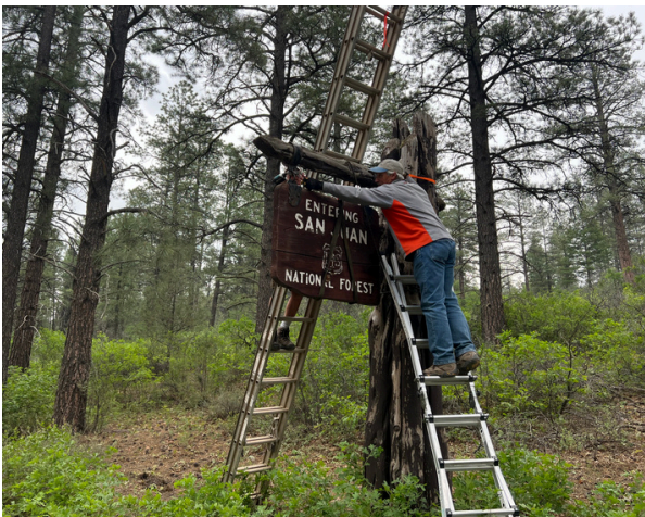
Removing sign hardware
