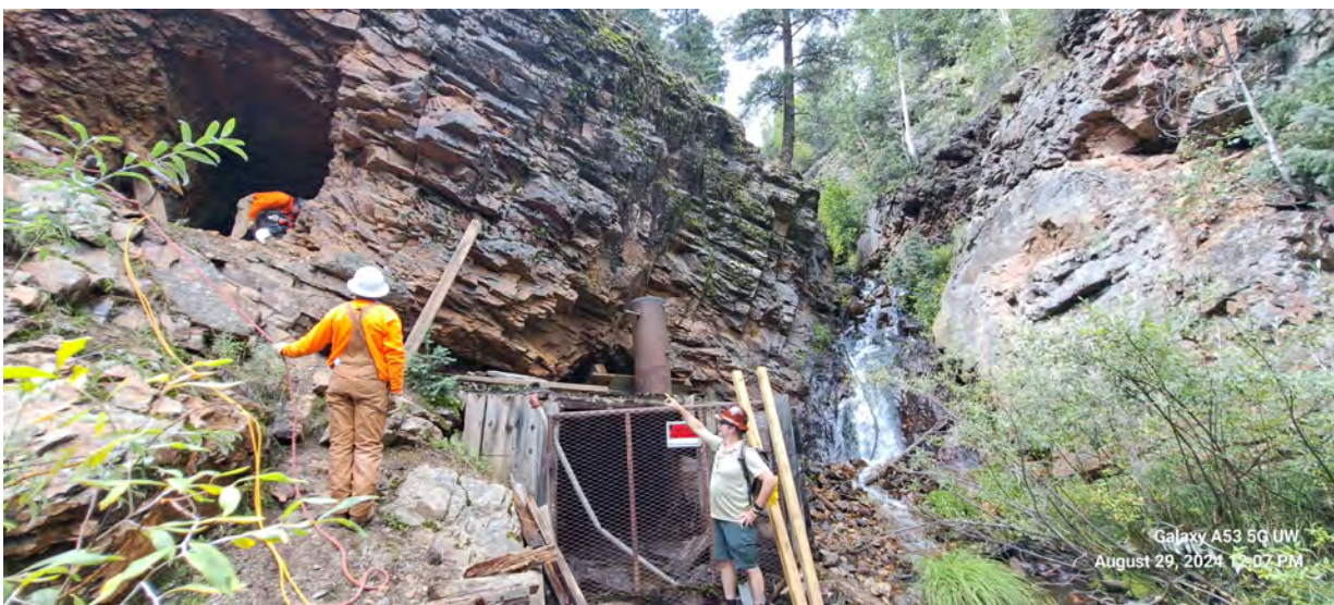
James Blair, SJNF Geologist discusses the mine closure with employees from High Country Solutions who were contracted to perform the closure. The lower opening is an attempt at restricting access installed by a miner some decades ago and was replaced by a secure entry with locking gate.
