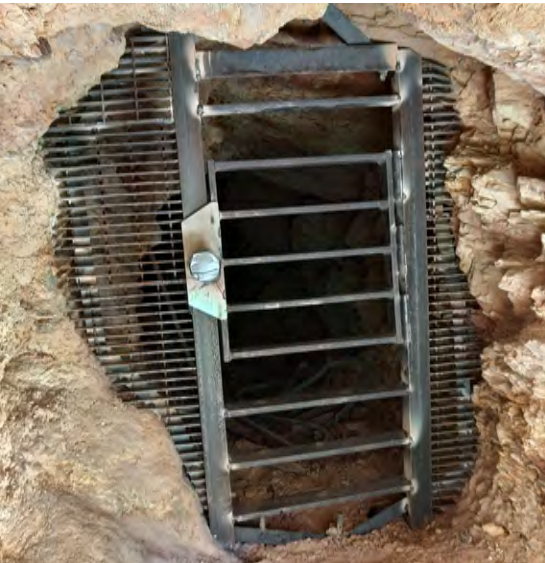
Adits post closure. The closures are designed to keep unauthorized people out, while providing access to the adit for bats.
