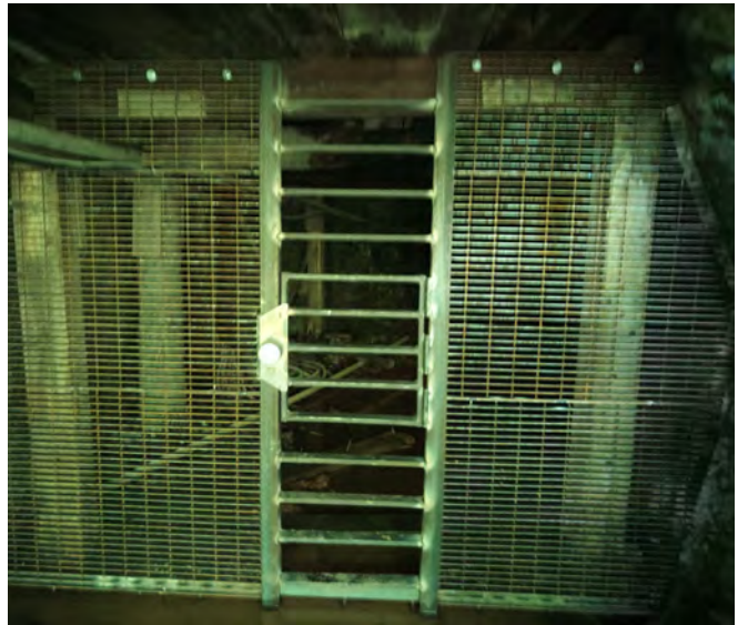
Adits post closure. The closures are designed to keep unauthorized people out, while providing access to the adit for bats.
