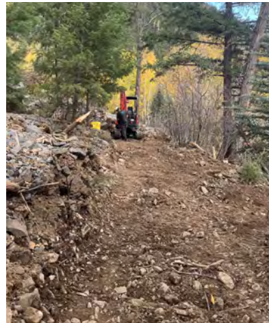
The mini-excavator accomplished in a handful of days what would have taken hand crews weeks
