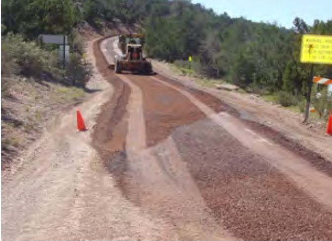
View of NFSR 249 during aggregate placement
