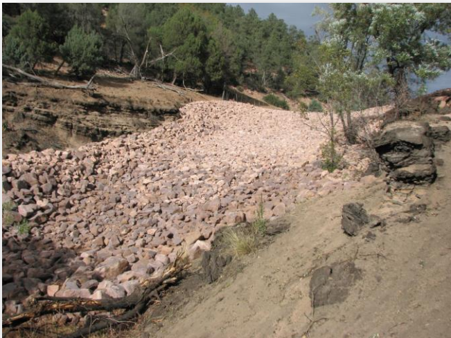
Profile view of area filled to restore channel gradient and arrest the head cut
