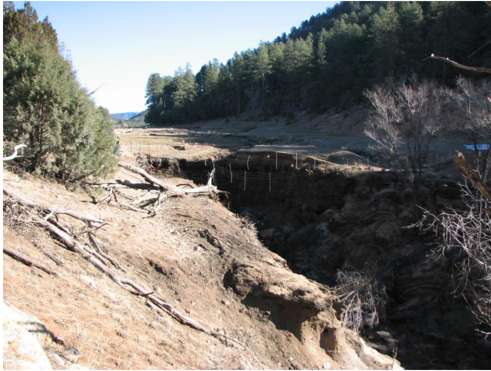
View of head cut prior to restoration in 2011 (looking upstream)
