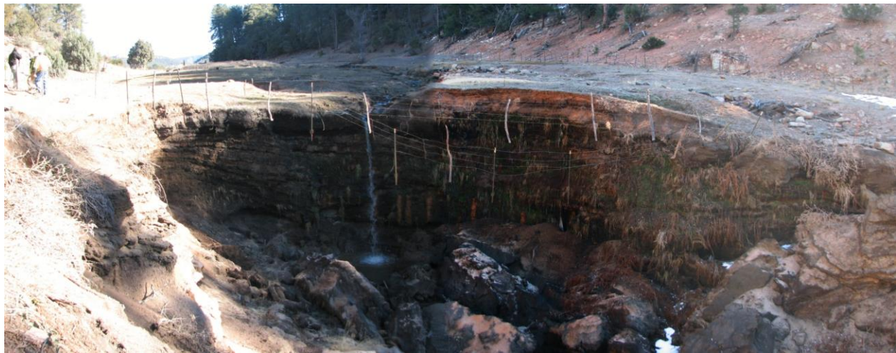
View of head cut prior to restoration in 2011 (looking upstream)
