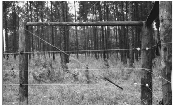
**Energized high tensile wire fence will withstand falling debris. Strategically locate power switches to improve pasture access and diagnosing power failures.**
