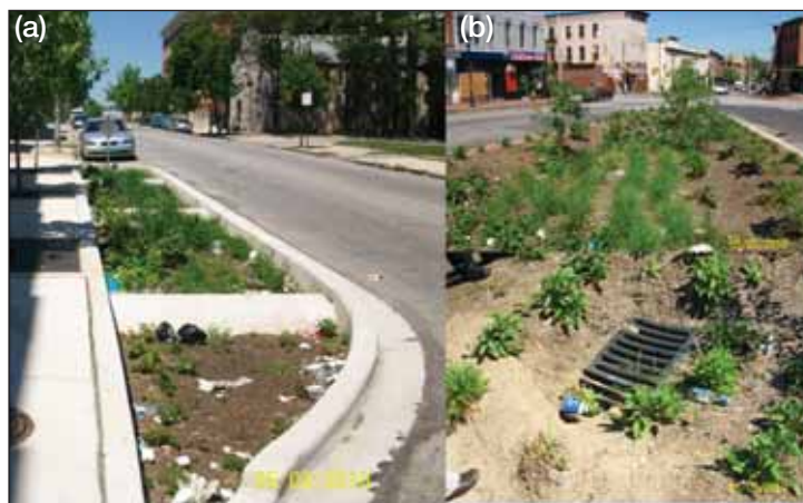
Figure 2. Examples of advanced bio-infiltration projects established in the Baltimore Street subwatershed of WS263. Photos show (a) curb extension with three underground tree boxes and (b) bioretention BMP installations. Total costs for the curb extension installation were over $79 000, including over $16 000 for design. Total costs for the bioretention installation were over $170 000 and included over $38 000 for design.
