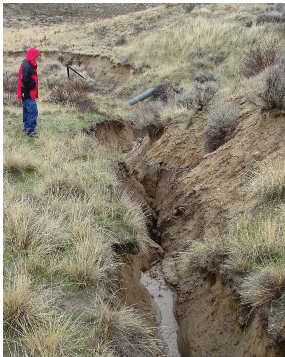
Figure 2. An active gully below a road drain point in the western United States (Photo credit: USDA Forest Service).
