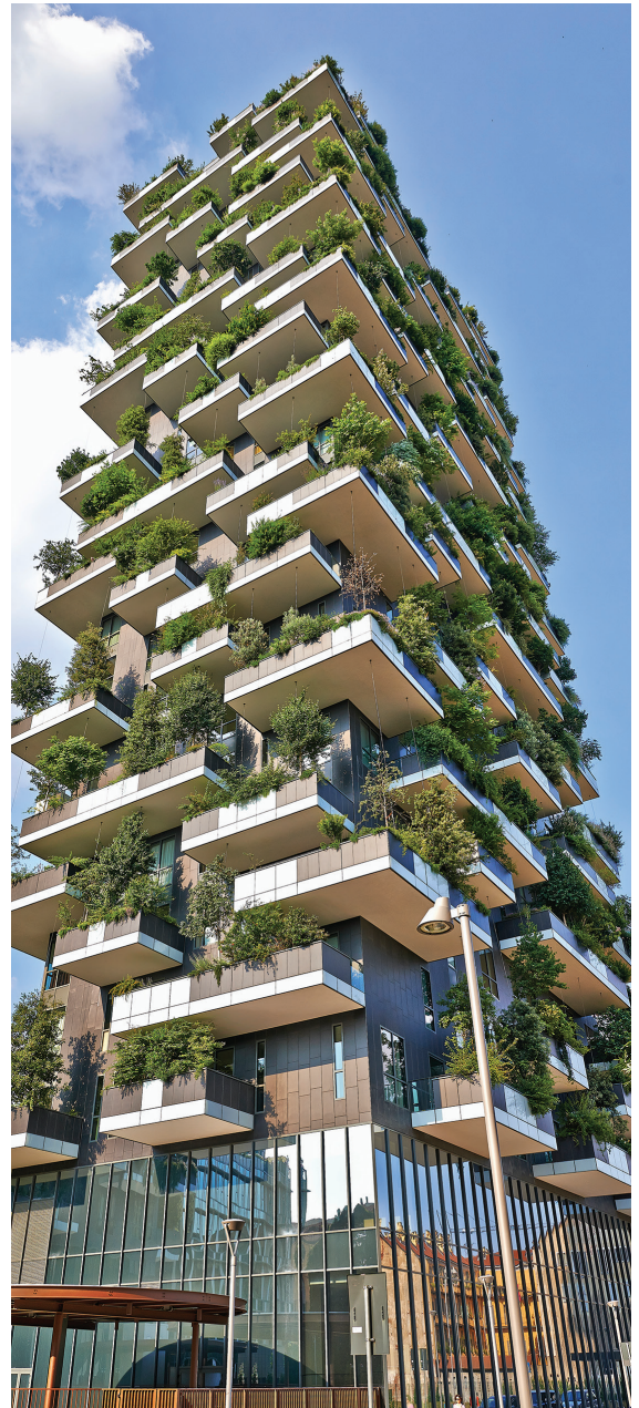
Bosco Verticale (Vertical Forest) is a pair of residential towers in the Porta Nuova district of Milan, Italy. Photo by Patrick Bombart, https://www.flickr.com/photos/capture-creation/23388324221 .
