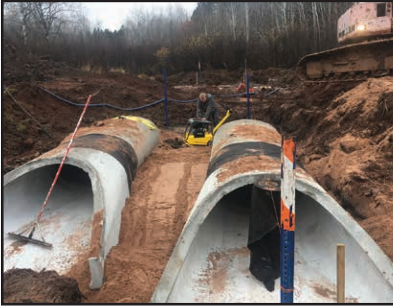
Bad River staff replacing a culvert on a tributary to Sucker Creek, which was regularly overtopped by water during spring floods. Funds were obtained through an EPA Great Lakes Restoration Initiative (GLRI) grant. (Photo by Eric Andrews, Bad River.)
