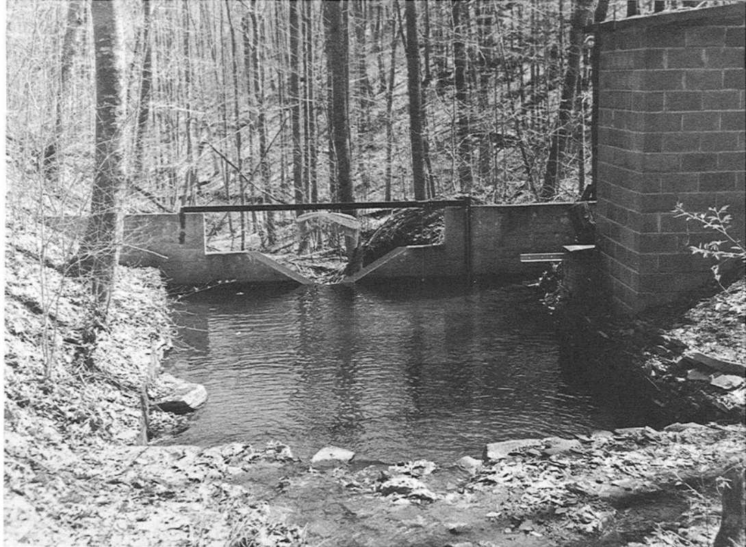
Figure 20.—A weir and gage house of the type used in watershed-management studies. This is a view from upstream.
