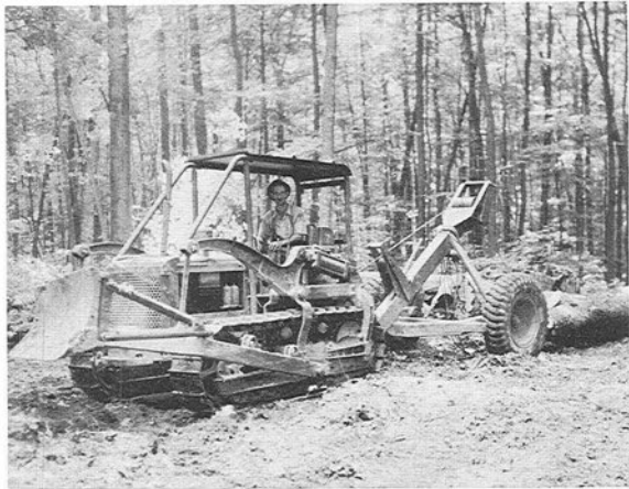
Figure 11.—The Fernow Forest personnel use a crawler tractor with a two-wheel arch to winch in and skid tree-length logs.
