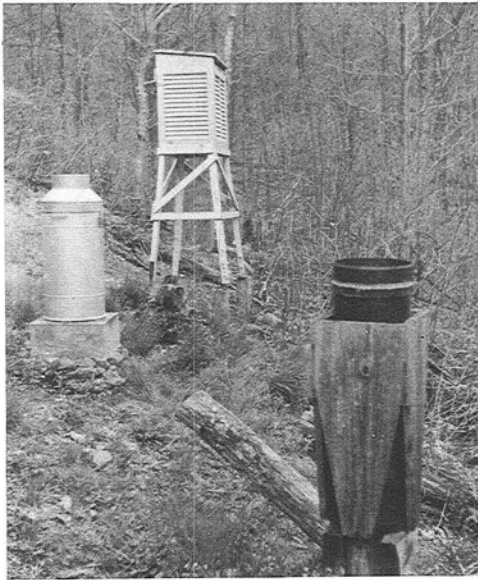
Figure 21.—Instrument installations used in watershed studies. Right foreground, a standard rain gage. Middle distance, left, a recording rain gage. Background, a weather-instrument shelter.
