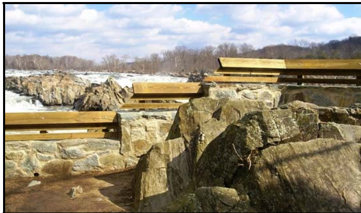
Recreation Fee funds improved visitor safety issues at Great Falls Park overlooks by providing guard railing.
