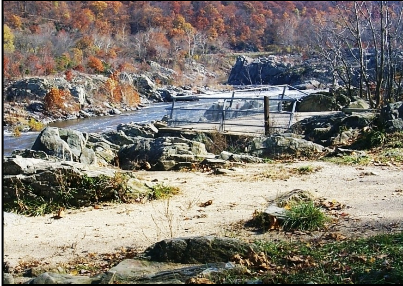
Prior to improvements, visitors often ventured off the designated path near this overlook at Great Falls Park, jeopardizing visitor safety and negatively impacting resources.
