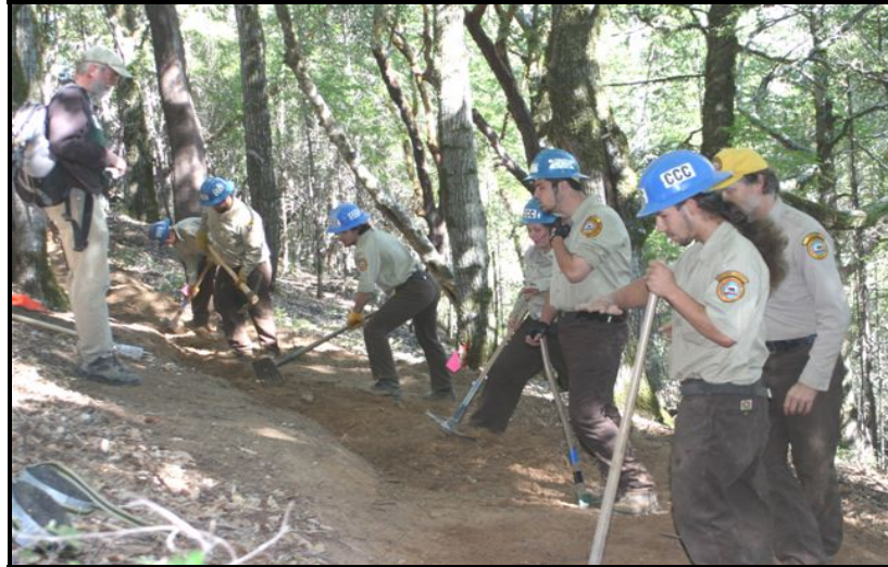
A California Conservation Corps crew and volunteers perform construction on a Mountain bike trail.
