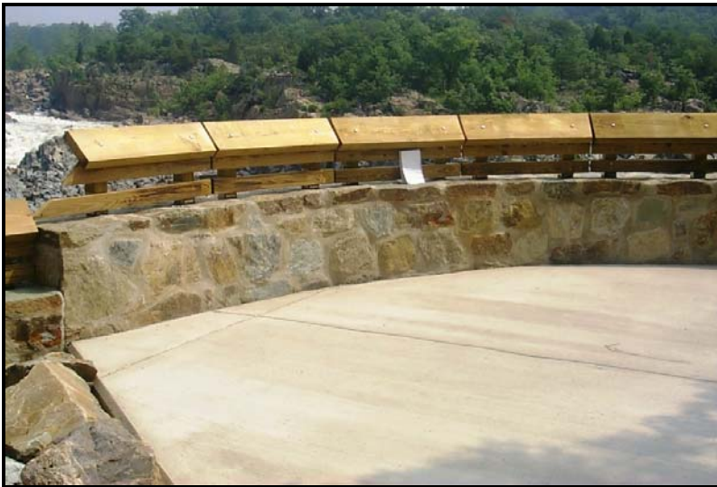
The completed new overlook, funded by Recreation Fee revenue, allows visitors to safely access and enjoy the same beautiful view while protecting resources.
