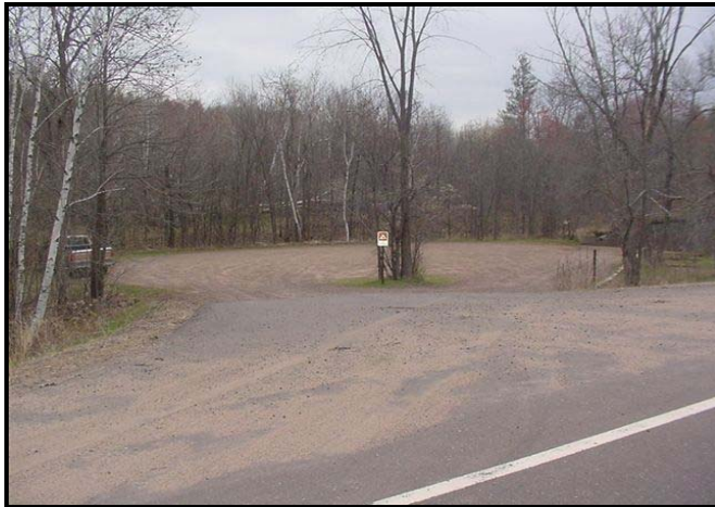
The gravel parking area at County "K" Landing of St. Croix National Scenic River was undersized and caused safety concerns.
