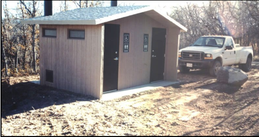
A new well was drilled at this site and now provides drinking water for the public and running water for the restrooms in the Henry Mountains, Utah.
