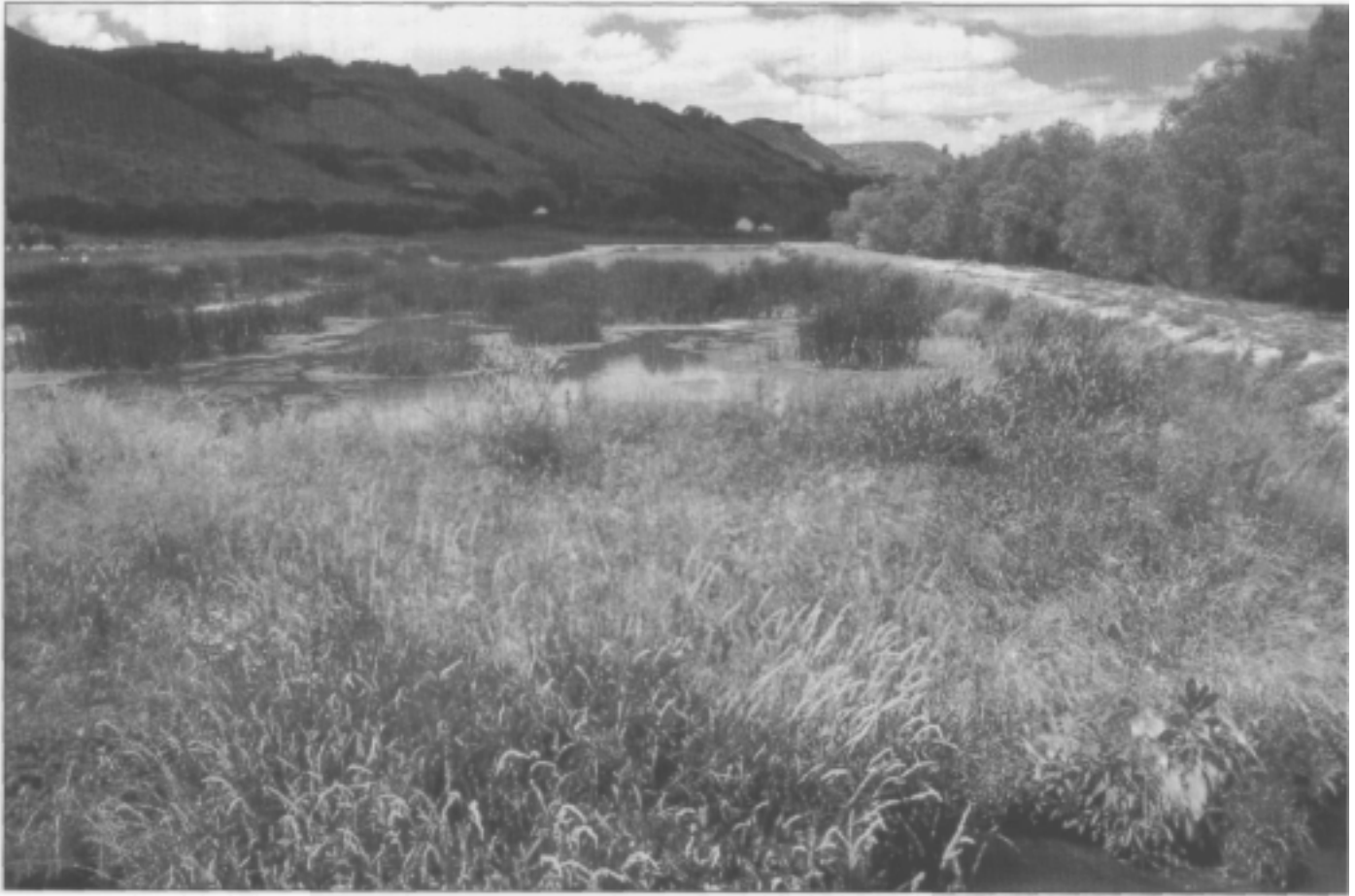
Figure 1. The Cedar Draw Water Quality Demonstration and Research Project located in southern Idaho 5 miles North of Buhl, ID (near the Snake River). This constructed wetland system is only 2 years old.
