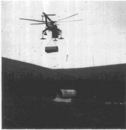
Military Sikorsky 5-64 sky-crane delivers fiberglass road matting used to stabilize vehicle trails on permafrost terrain in 1979. Note that the second mat on the ground is caught in the downdraft from the helicopter rotor. (Helmers collection)
