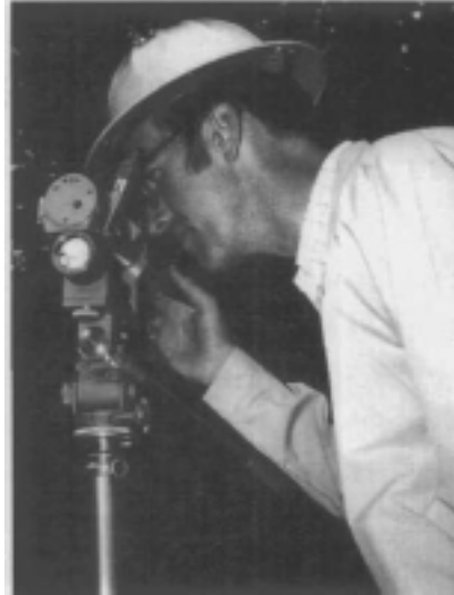
Research Mensurationist Bill Farr's long-term research in Alaska spanned the years from 1960 until his death in 1995 and laid the foundation for research alternatives for clearcutting. Here, he measures tree size and height with an optical dendrometer. (Juneau, unnumbered)
