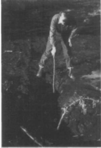
Charles Cushwa examines erosion on a tire line constructed over permafrost on the Wickersham Dome fire area northeast of Fairbanks in July 1971, less than one month after the burn. (Wright collection)
