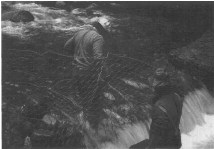
Construction of a gabion dam at East Creek on Young Bay Experimental Forest in 1969. (Swanston collection)
