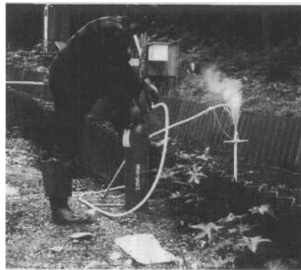
Bill Walkotten developing and testing a liquid CO 2 gravel sampler on the flume at Young Bay Experimental Forest in 1974. (Swanston Collection)
