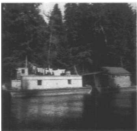
Boats and water routes provided access and a home-away-from-home for livid crews in Alaska. Research "wamgans," a name derived from the Ojibwa term "wannikan," meaning "man-made hole," were essentially barges with living quarters and laboratory facilities constructed on deck that were towed to field sites. This one anchored on Harris River in 1958. (Juneau 854)
