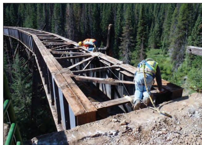
Figure 19—The Route of the Olympian project involves trestle and tunnel repairs that required an engineering assessment and design plan, highly technical construction expertise, and specialized heavy equipment.
