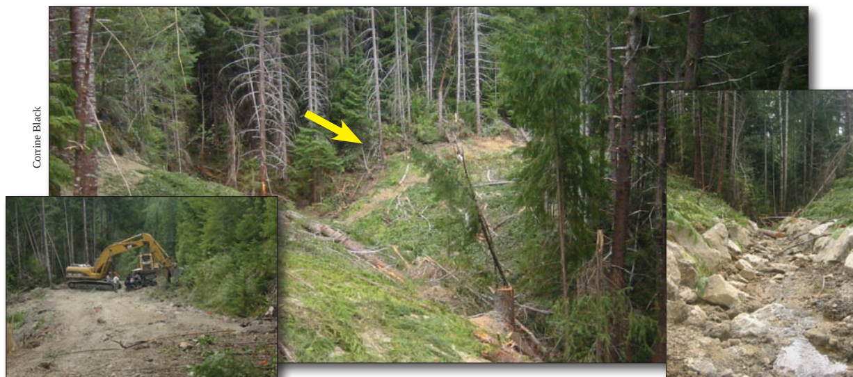
Left photo: Karuk Tribes restoration crews marked the limit of excavation and reviewed site plans prior to decommissioning this perennial stream crossing in the Bluff Creek watershed. Middle photo: View of completed work. The arrow marks the spot where the left photo was taken. Right photo: Closeup view of newly excavated stream channel.
