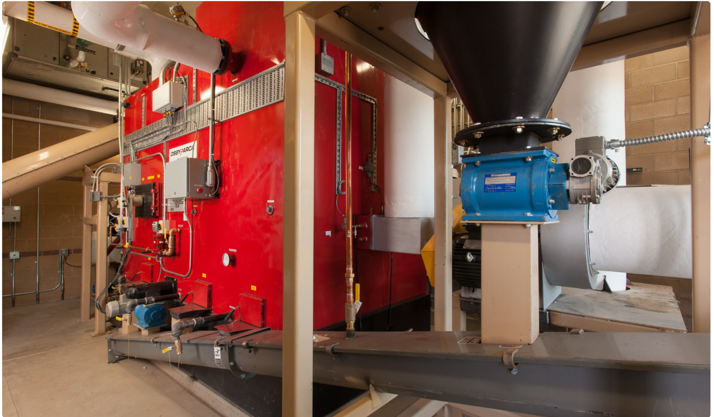
3.5 MMBtu/hr wood chip boiler system, $500,000 capital investment, South Park School, Fairplay, Colorado – completed in 2012.
