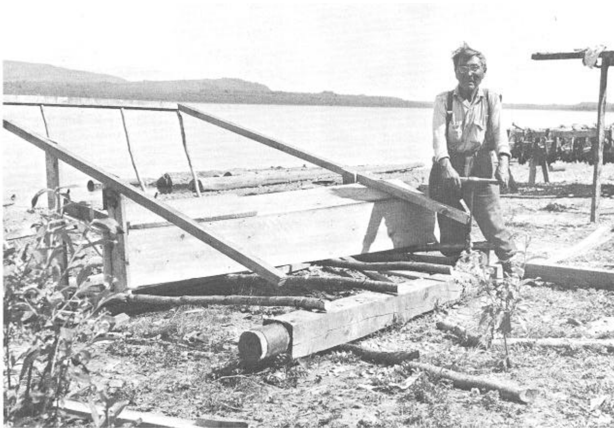
Figure 32.--This resident of Aniak on the lower Kuskokwim River is building a fish wheel from materials obtained locally--a few boards from a local sawmill and saplings from along the river.
