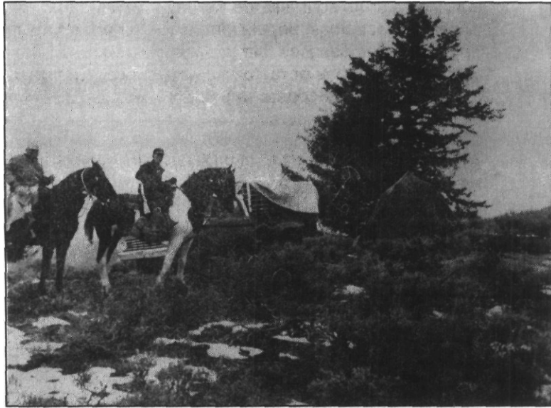
Figure 5-3 Recreation use of the program area includes camping, fishing, hunting, rock collecting, bird watching and others. Completion of developed recreational sites has proved difficult because of water and sanitation problems, and costs of maintenance and garbage collection.
