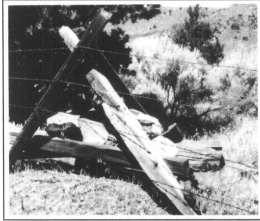
Figure 12—"Rock jacks" and "cribs" are used where the soil is too rocky for post holes: (A) "Rock jack" made of six split juniper posts. (B) "Crib" made of treated pine posts and boards. Juniper posts are often used in "cribs."
