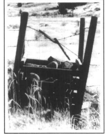
Figure 12—"Rock jacks" and "cribs" are used where the soil is too rocky for post holes: (A) "Rock jack" made of six split juniper posts. (B) "Crib" made of treated pine posts and boards. Juniper posts are often used in "cribs."
