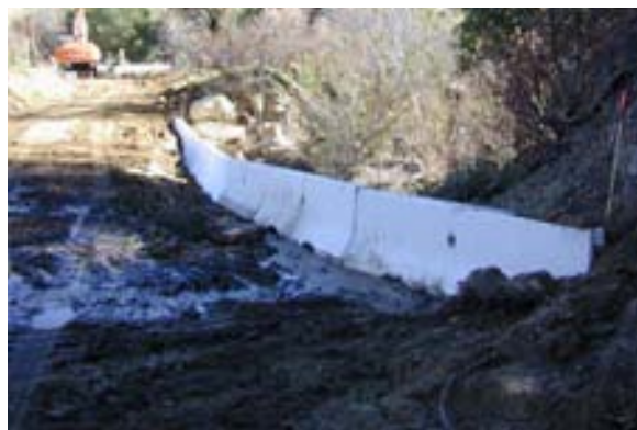
Fig. 4.24. K-rails installed at mile point 1.4.
