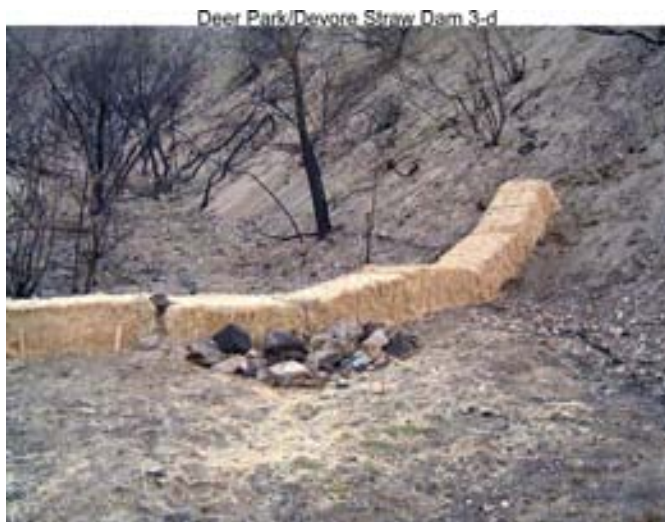
Fig. 3.54. Deer Park/Devore straw dam 3d viewed on 12-3-2003 installed in upper main channel. Note riprap below dam.
