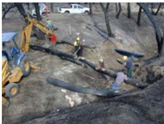
Fig. 4.9. Installation of log check dams begins.
