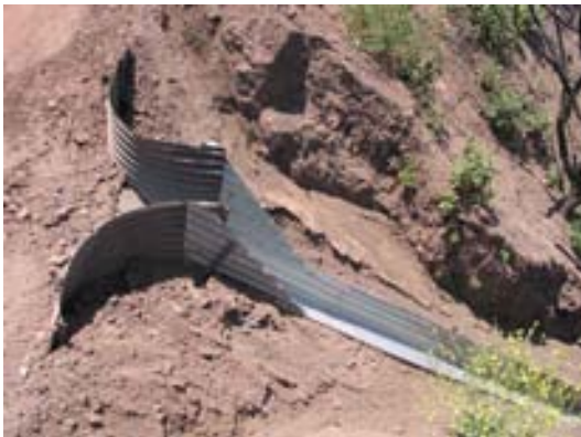
Fig. 4.36. Inlet side of overseide drain (mile point 4.1 – Ranger Station to Dough flat)
