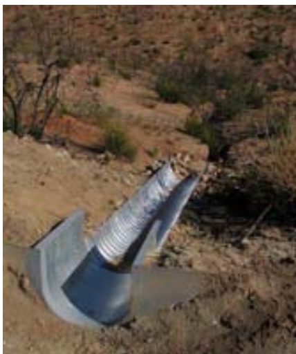
Fig. 2.41. New upside drain with extension and riprap installed on West Side Truck Trail. Mile point 0.6, photo #100-0038.
