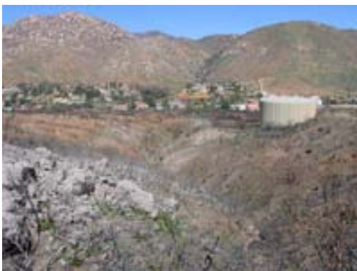
Fig. 2.30. View looking downslope to water tank of main channel. Photo # 100-0032 taken on Mar 24, 2004.
