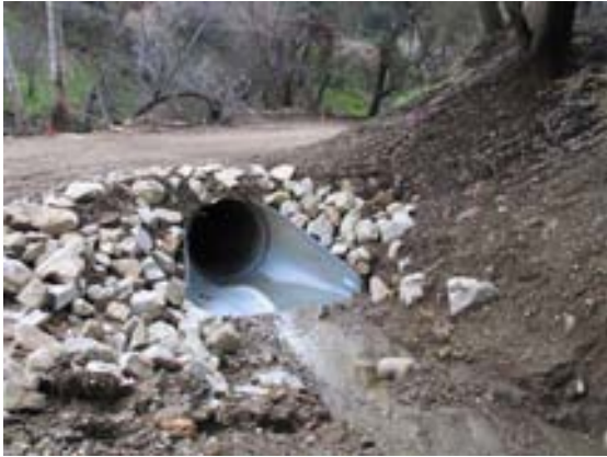
Fig. 4.28. New culvert with rock armoring at inlet (mile point 1.97)
