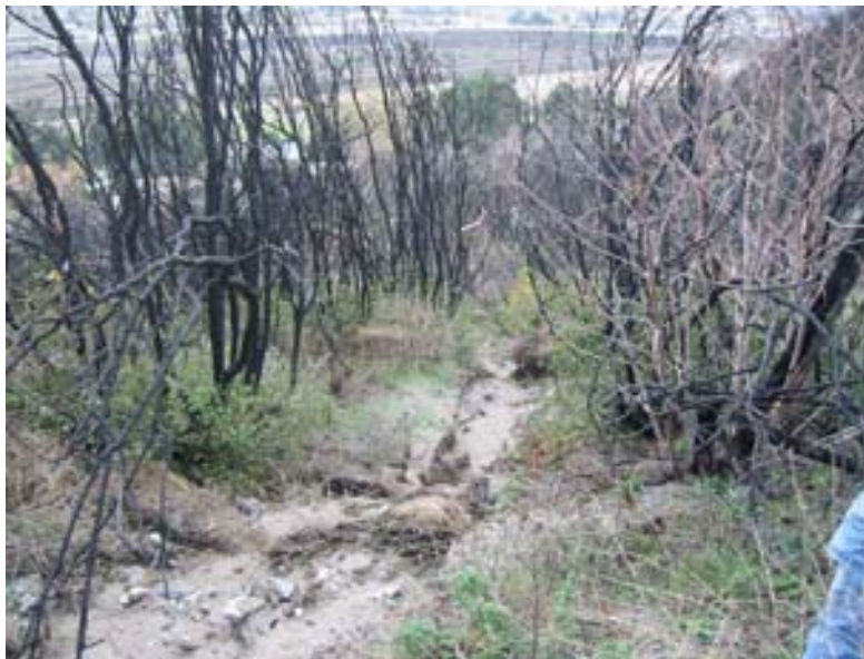
Fig. 3.60. Blowouts of side channel check dams also occurred in the October, 2004 storm events.
