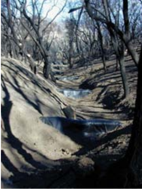
Fig. 4.11. Finished log erosion barriers viewed up channel.
