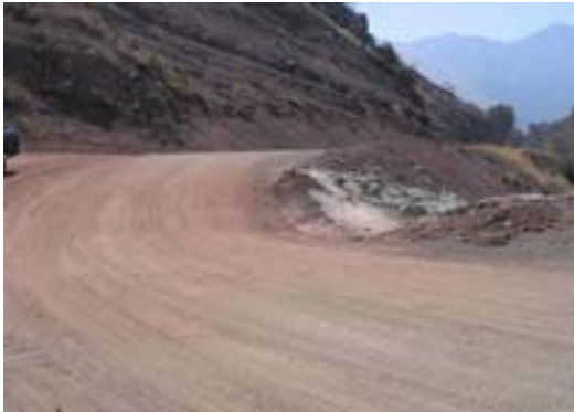
Fig. 4.35. Low water crossing with Big Mac (mile point 0.6 – Ranger Stn to Dough Flat.
