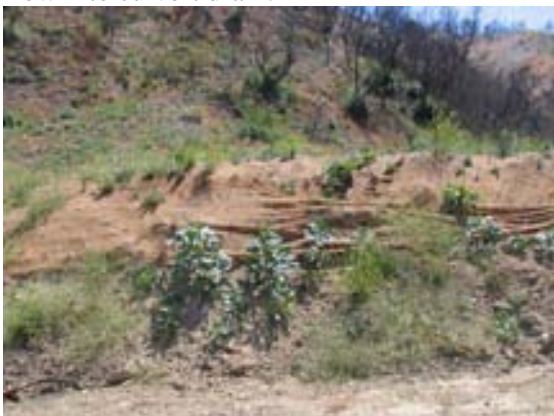
Fig. 4.30. Geo-textile fabric with jute was added on slope bordering road located above the 60 in. culvert (mile point 2.1).
