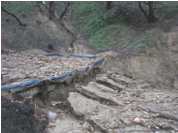
Fig. 4.14. Cutting back under the log check Dam.
