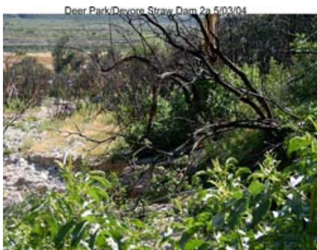
Fig. 3.47. Deer Park/Devore straw dam 2a viewed on 5-3-2004. Note vegetation growth on stored sediment.
