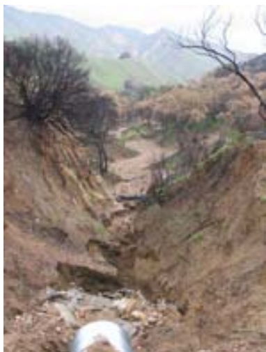
Fig. A.11. Outlet of culvert looking into drainage
