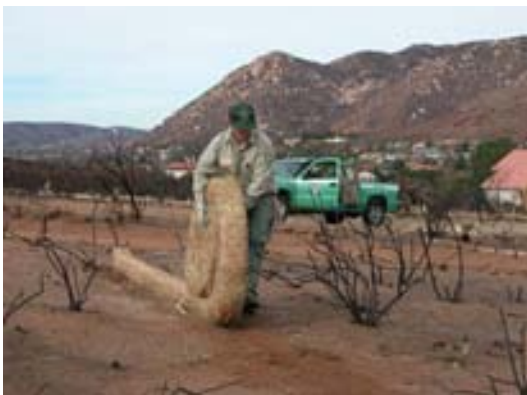
Fig. A.3. Fiber roll being placed into trench.
