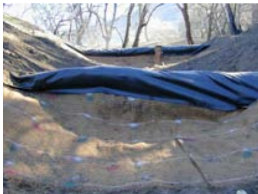
Fig. 4.10. Geo-textile fabric being spread over log check dam and fabric laid out below dam to act as an energy dissipater.
