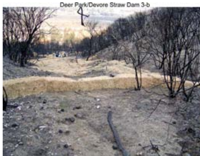
Fig. 3.51. Deer Park/Devore straw dam 3b viewed on 12-3-2003 immediately after installation in main channel.
