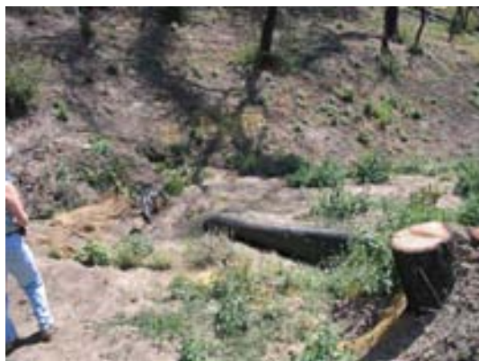
Fig. 4.21. To remediate the check dam installation, notching or removal of middle portion of some check dams was initiated.
