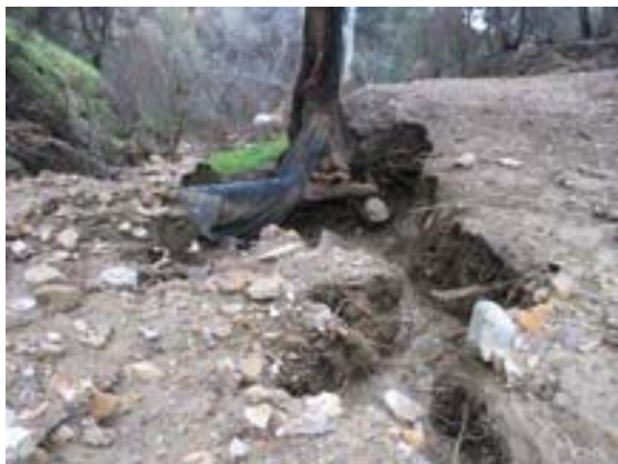
Fig. 4.15. New channel formed in newly deposited sediment causing check dam to fail at end.
