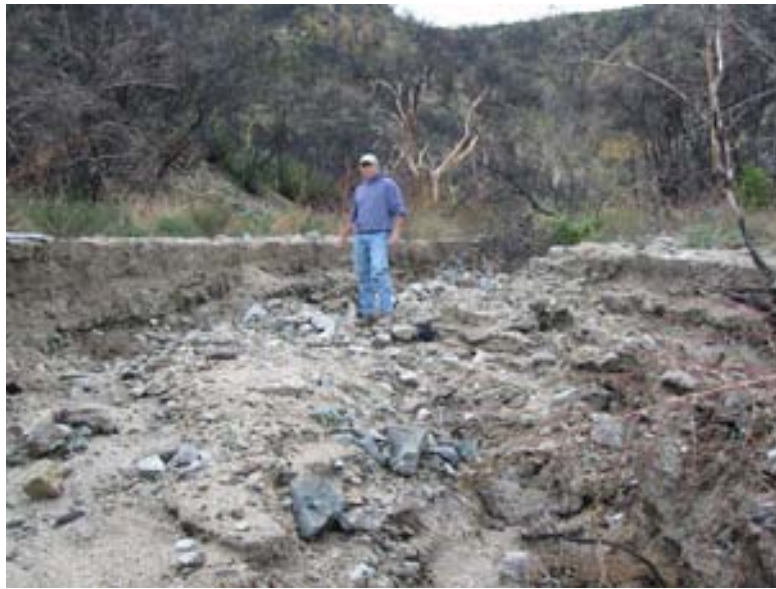
Fig. 3.59. Sediment was stored to the level of the cut banks. Sediment storage can be seen in Figs. 3.52 and 3.53. All of this material was released during the October, 2004 storm events when the check dam failed.
