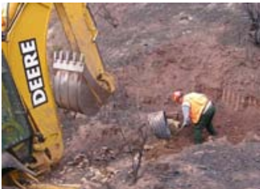
Fig. 4.32. Culvert being replaced.
