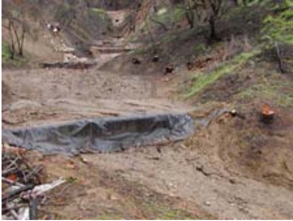
Fig. 4.13. Storage area behind dams filled to capacity.
