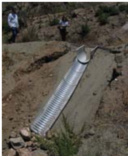
Fig. 2.33. New overside drain with extension at mile point 0.6, photo #100-0008.
