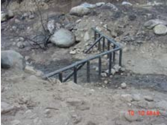
Fig. 5.4. Installation of a trash rack in Stoddard Canyon.
