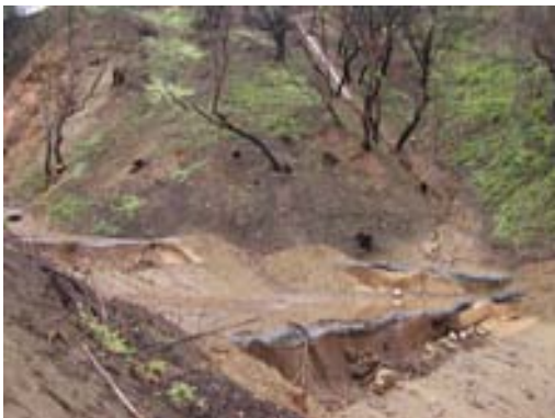
Fig. A.10. Water ponding behind check dam.
