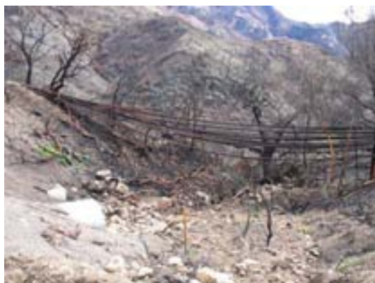
Fig. 4.2. Oil pipelines suspended across drainage in the Sespe area. The fire uncovered a vast array of functioning and non-functioning pipelines in the area. It was suggested that the pipelines be mapped and noted as working or not.
