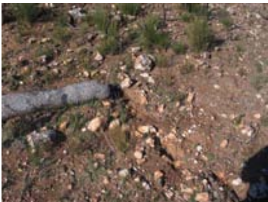
Fig. 2.26. Fiber roll incorrectly down-turned at end. A rill is beginning to form at the end where water is being channeled.
