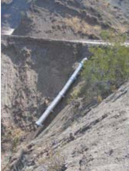
Fig. 4.34. Overside drain with extension (mile point 2.62 Squaw Flat Rd)
