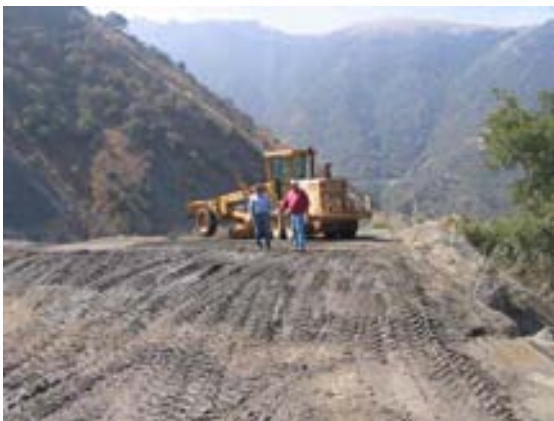
Fig. 4.33. Road grading completed and approximately 280 cu. yds of mud, rock, and debris was removed at mile point 1.9.
