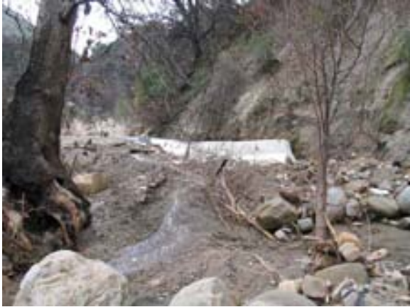
Fig. 4.25. Drainage entering the road
