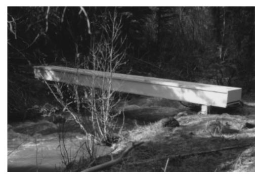
**Figure 6**—Platform (3 x 24 feet) resting on sill at Silver Creek, near Wolf Creek Pass, CO.
