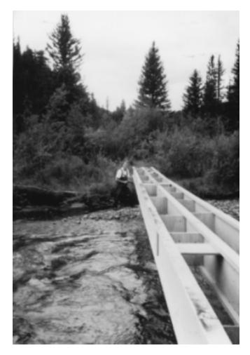
**Figure 5**—Plywood rectangles are used as spacers on this 3 x 60 foot platform on South Fork Cache la Poudre, near Fort Collins, CO.
