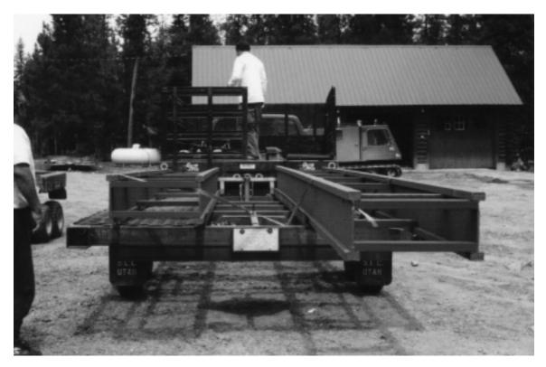
**Figure 4**—An example of platform frames constructed using 2 x 4 lumber as spacers. Most of the construction for smaller platforms (15 and 24 feet shown here) can be done off-site because the frames are light enough to be carried to the site by two to three persons.
