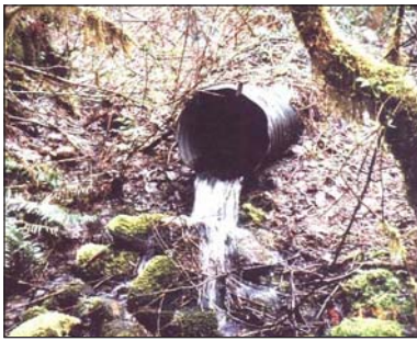
Pretreatment: fish passage barrier at small culvert site.
